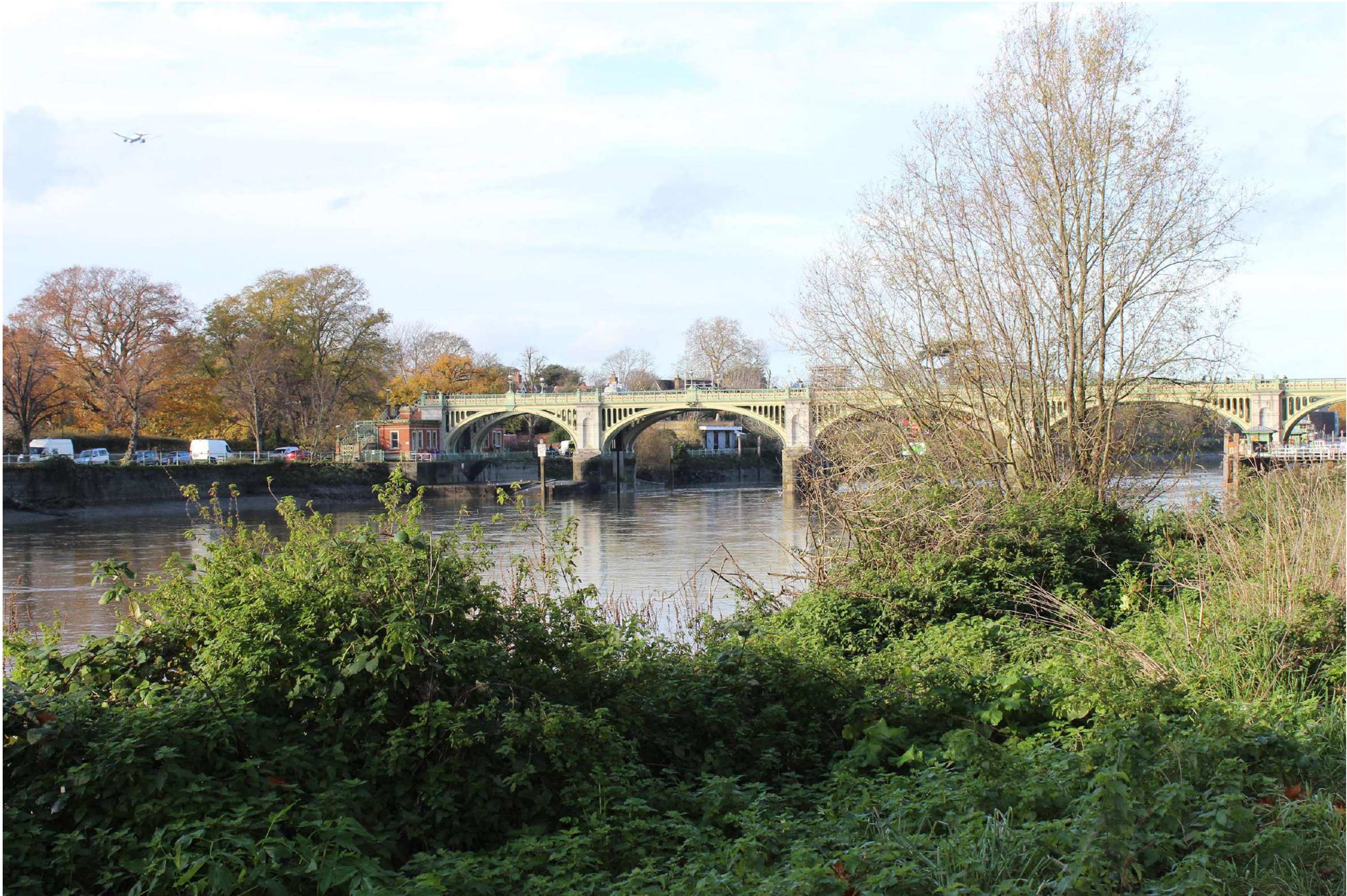
Existing View 07 - 28/11/22 – 13:30pm
