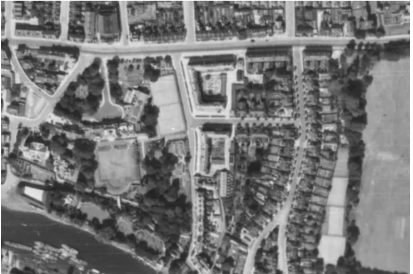
An extract of a 1944 aerial photo showing the garages in situ. © Historic England raf_106g_la_29_rs_4115
