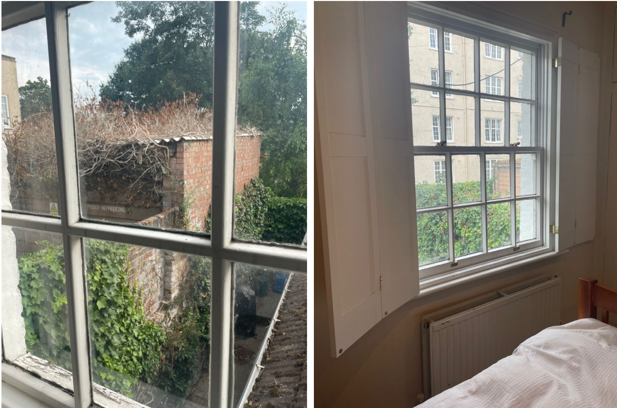
Image: View from rear window (left) and front window (right)
