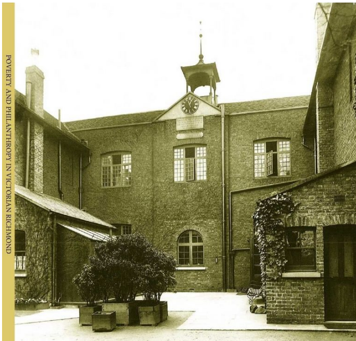
Figure 3 Front elevation of building, 20th century
