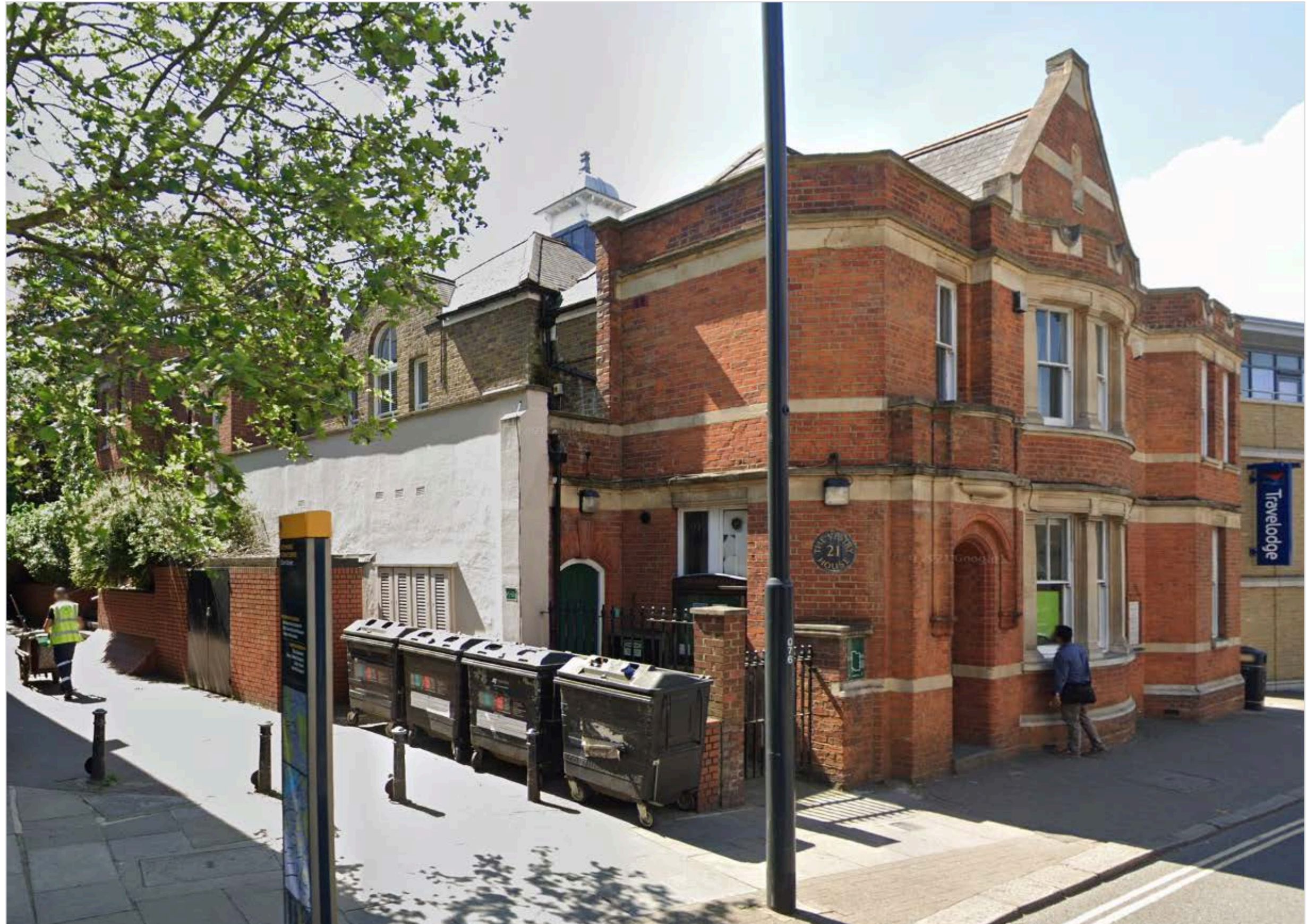
Corner of east and north elevations of Vestry House, viewed from Paradise Road.
