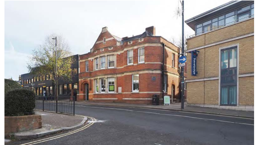
North elevation of Vestry House, facing Paradise Road.
