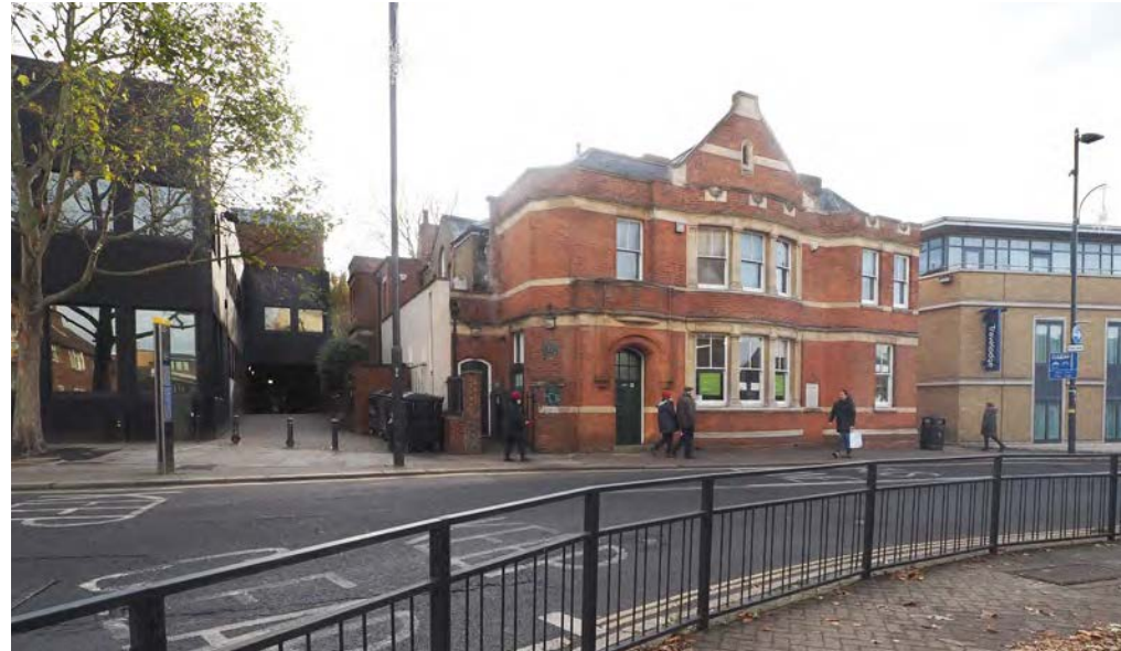
North elevation of Vestry House, facing Paradise Road.
