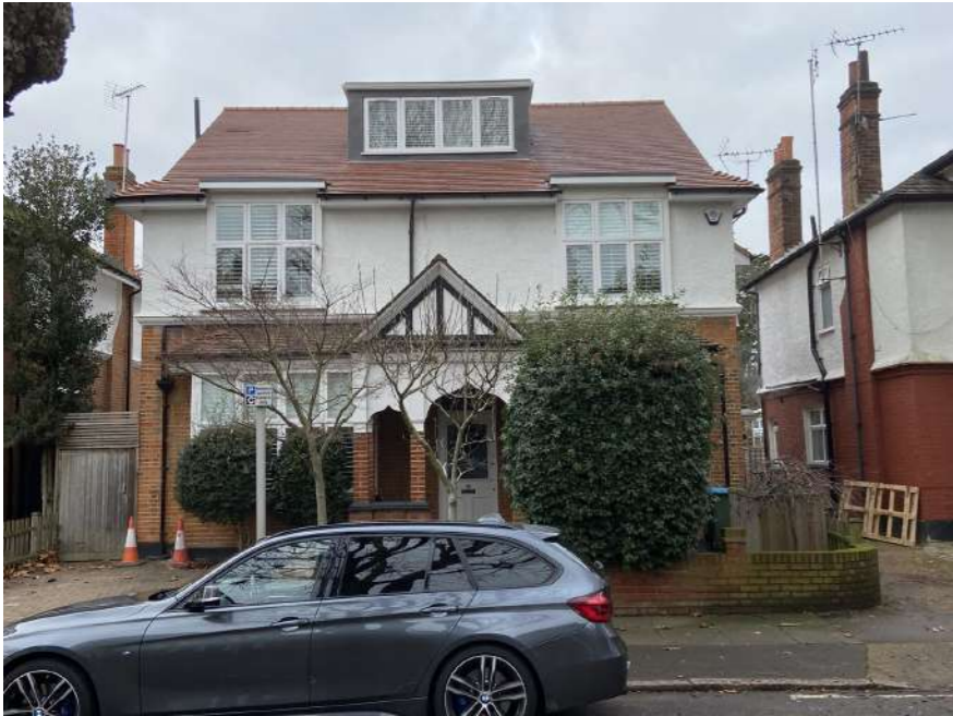
Front elevation of number 19 Cole Park, neighbouring the application site.
