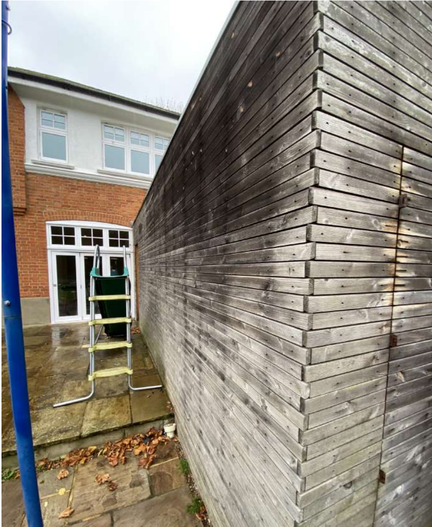
Timber cladding to the existing store room extension.
