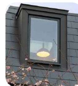
Zinc clad dormer window with a slim framed aluminium window
