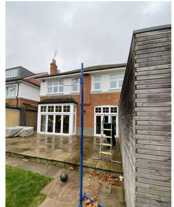
View of the rear elevation.
