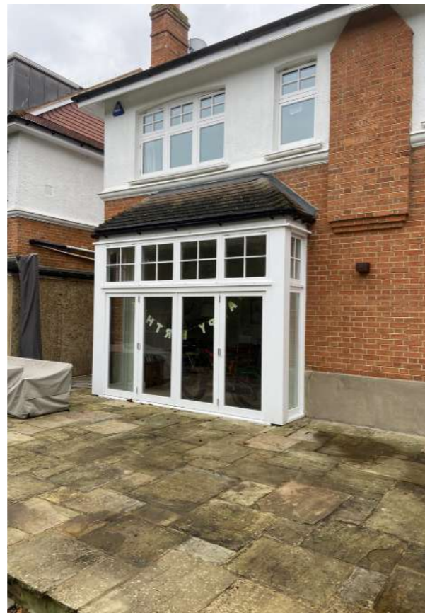
View of existing bifold doors to rear elevation to be retained.
