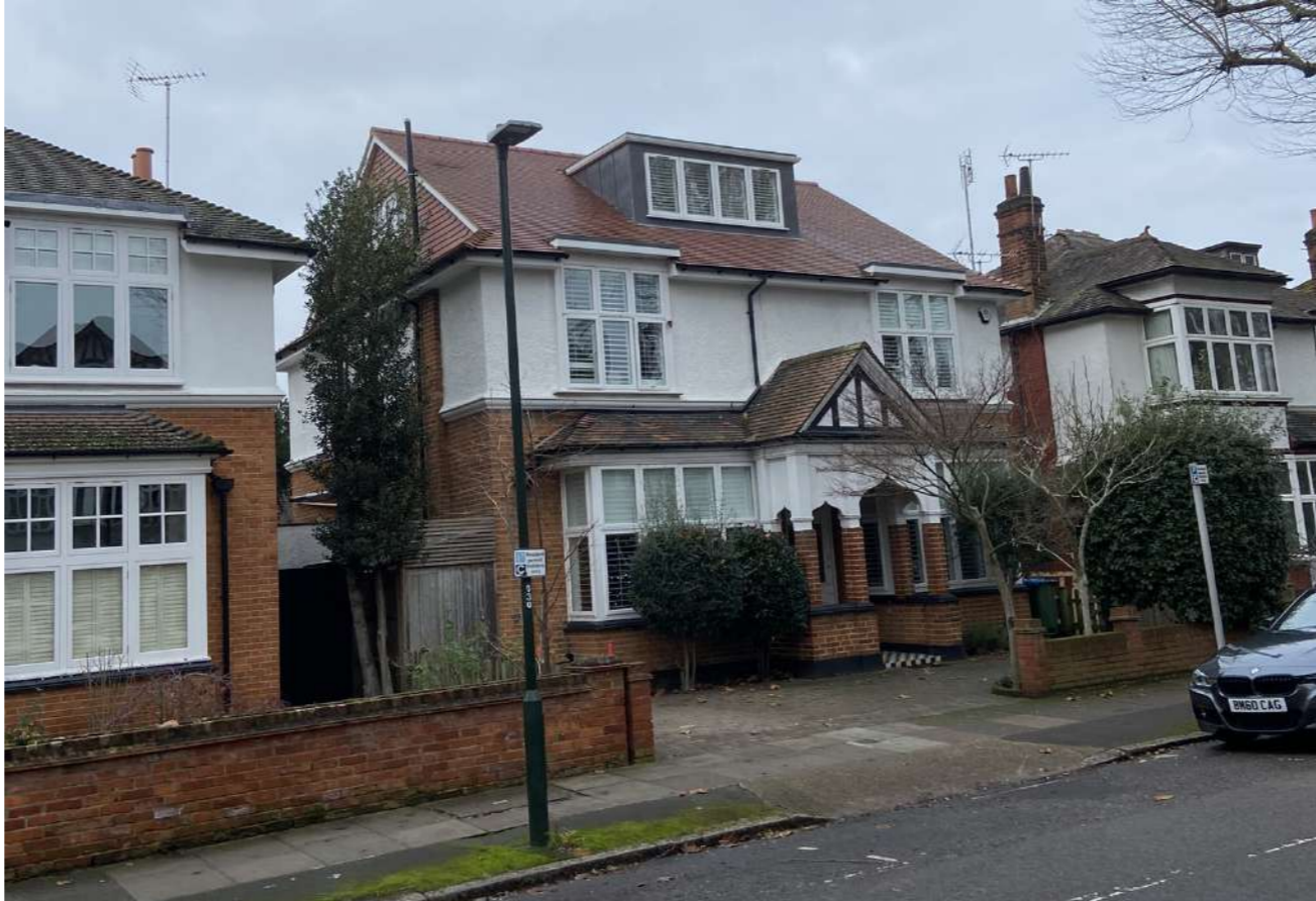
Front elevation of number 19 Cole Park, neighbouring the application site, incorporating a loft extension with gable ends and a dormer window to the front elevation. 17 Cole Park shown on the left of the image.
