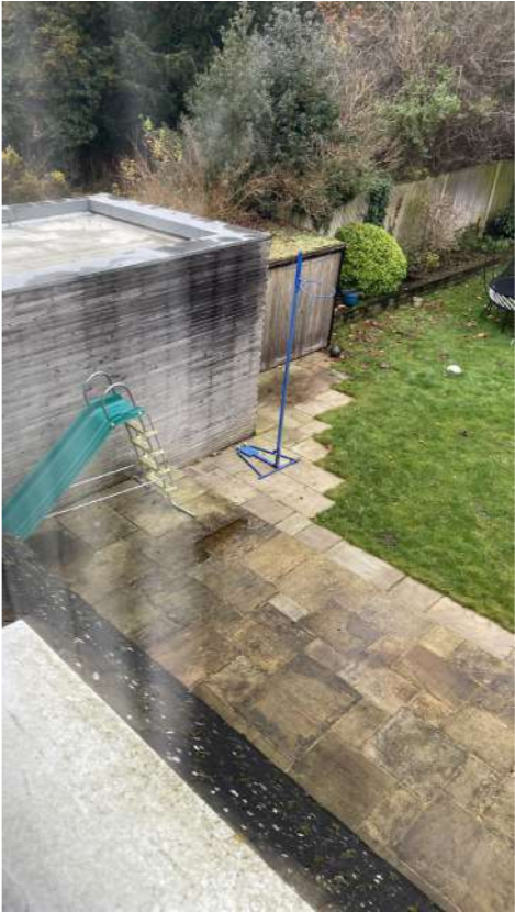
Existing timber clad extension viewed from the first floor of number 17 towards number 15.
