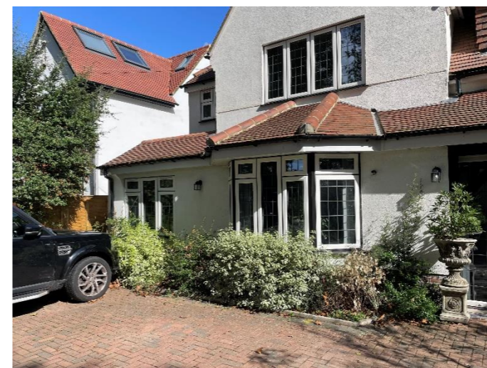
Fig 9 The front elevation and neighbour (No. 76)
