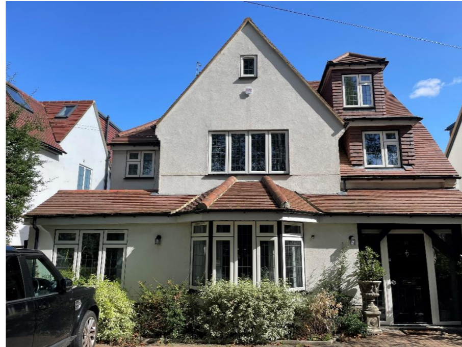
Fig 2 / Showing the front elevation of the detached property
