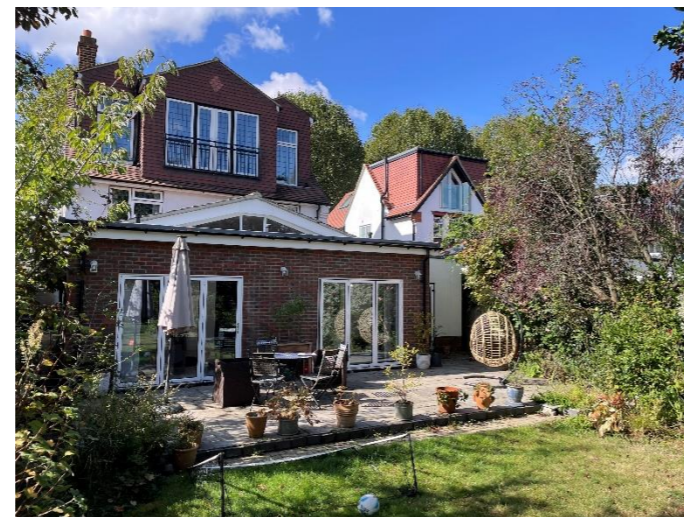
Fig 8 The rear elevation and neighbour (No. 76)
