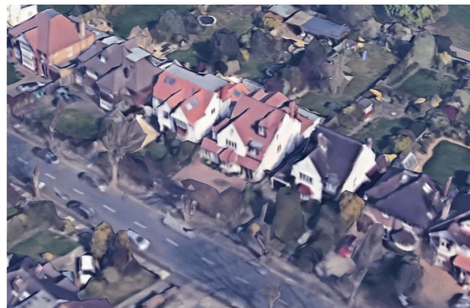
Fig 3 / This aerial photo illustrates the setting of the building toward the south-west end of the home.
