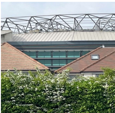
Figure 19. View from Across A316 of 9 and 11A&B T Ave
