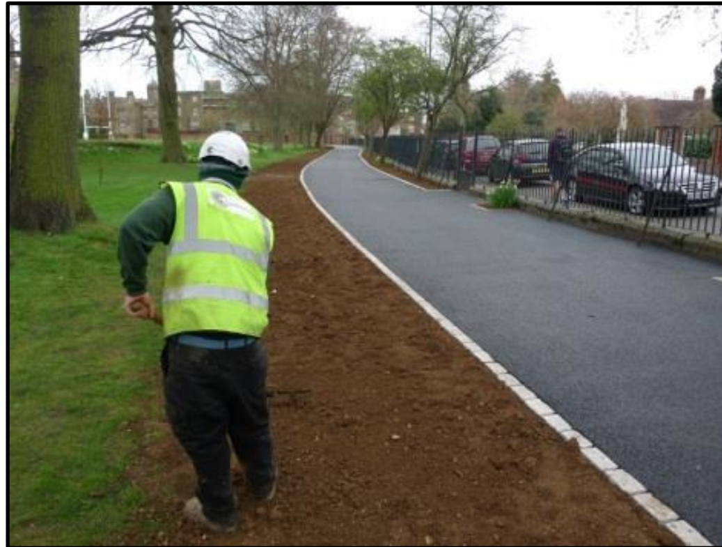
Fig 15 – All 'making good' topsoil will be BS3882 compliant and raked out by hand to no greater depth than 100mm.
