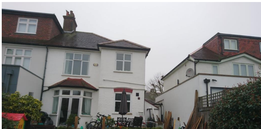
Rear of No. 24, 22 and 20 (right) showing scale of neighbouring extensions
