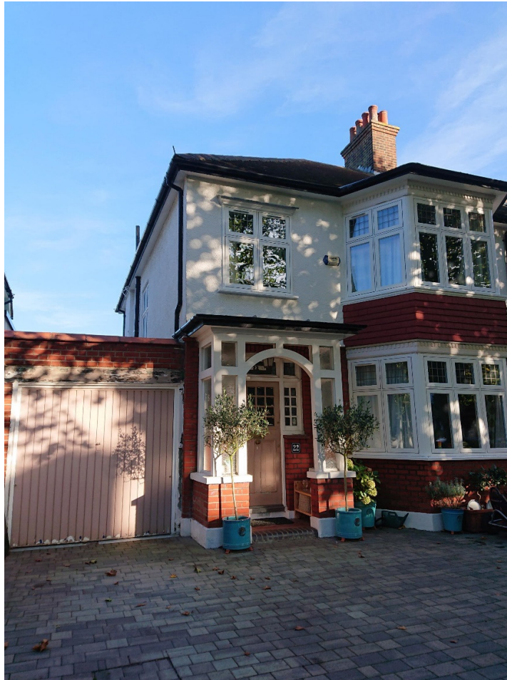
22 Park Drive, Front Elevation (Client photo, 15/10/2023)
