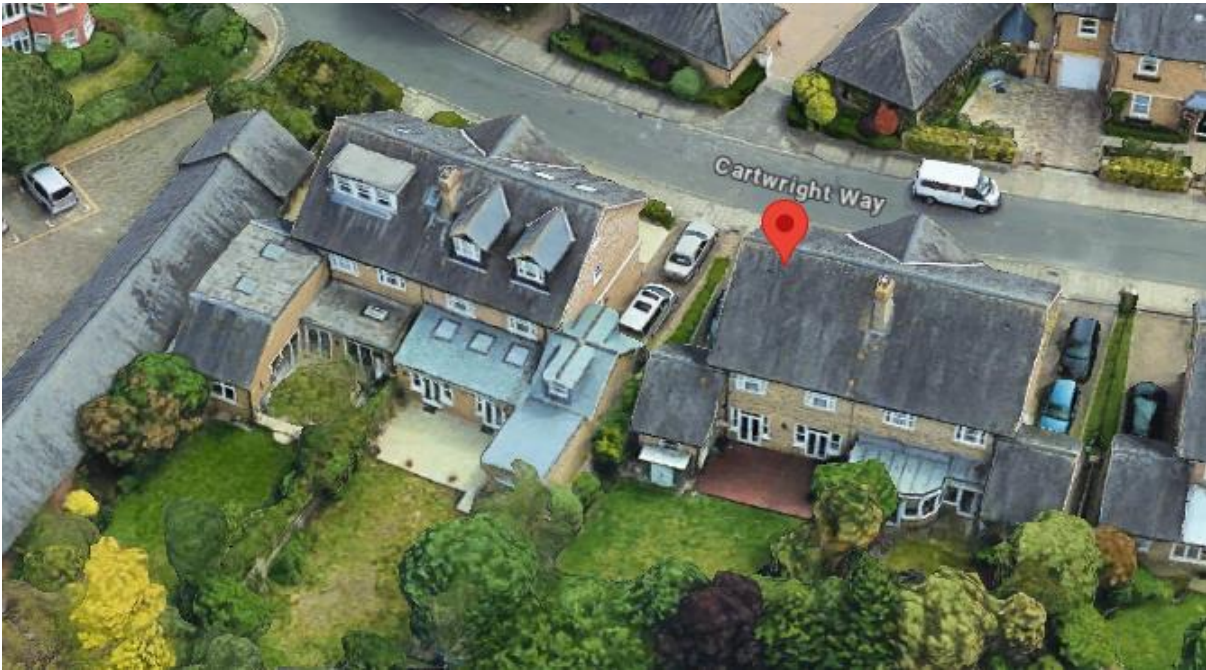
Figure 6 – Aerial photographs of immediate locality
