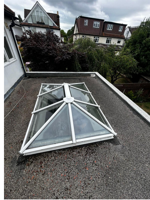
View towards Fairfax Road
