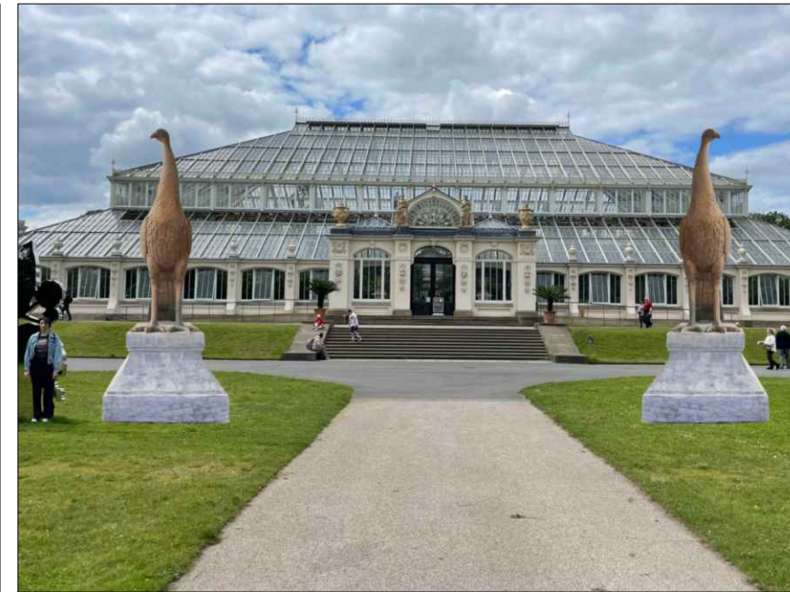
NORTH WEST VIEW FROM PAGODA VISTA
