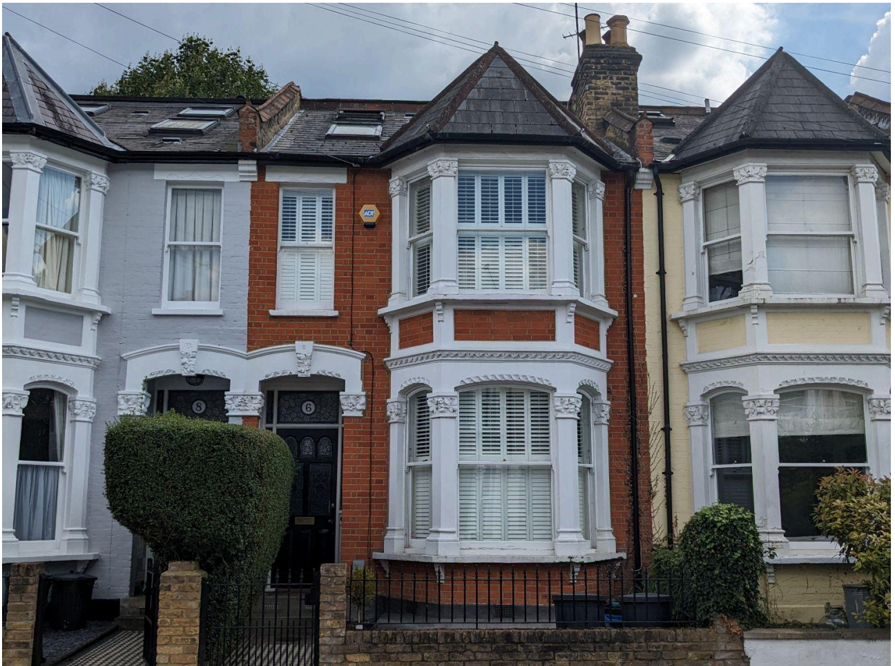
Figure 1: Photograph of building frontage.
