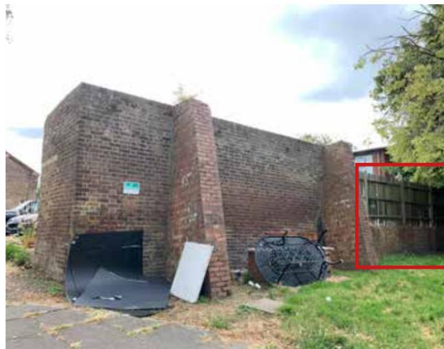
Figure 3.50 The rear elevation of the surviving section of garden wall, showing the modern buttressing. The south returning end of the wall (right) has been rebuilt using modern brick and fencing. This section of wall (also highlighted in red) will be rebuilt using material from the surviving north end of the wall
