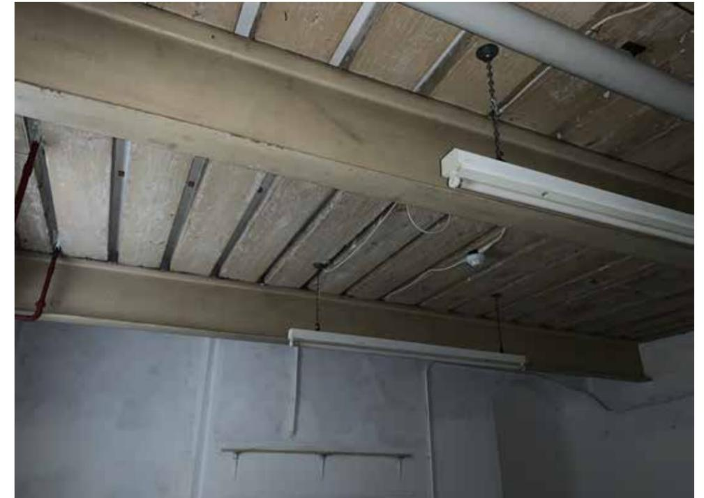
Figure 4.7 Modern ceiling beams and joists have been introduced in many rooms within the basement and replace historic features
