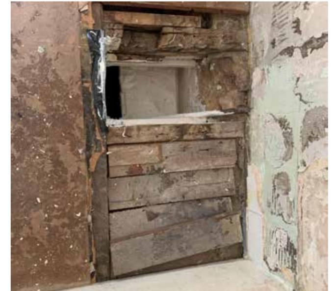
Figure 5.19 Photograph of exposed historic floorboards within the Meeting Room at Ground Floor Level
