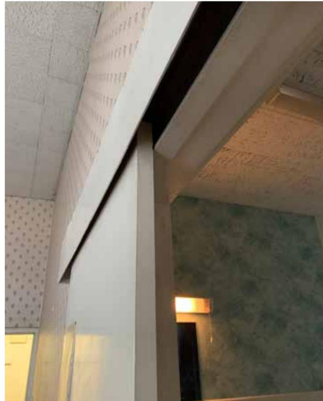
Figure 4.18 An example of the many modern partition walls introduced to subdivide historic spaces in the building. Modern dropped ceilings have also commonly been installed. The room in the photograph has been created through the subdivision of the former Vice Principal's bedroom and sitting room
