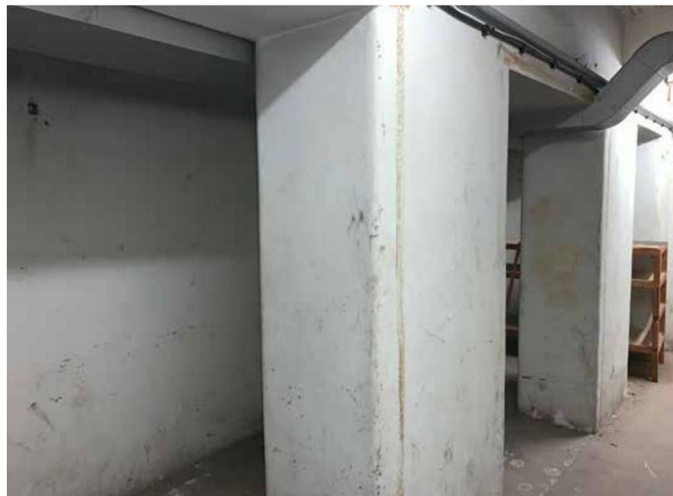
Figure 4.6 Early nineteenth-century supportive columns in the basement. Modern MEP equipment has been inappropriately fitted here.
