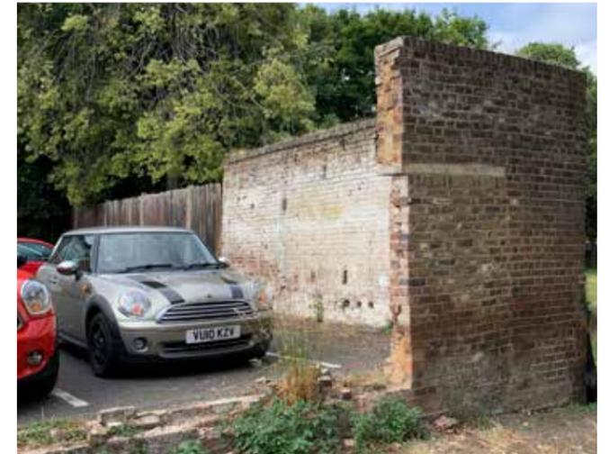
Figure 3.46 Photograph of the surviving section of garden wall. The wall is in a state of disrepair and is structurally unstable.
