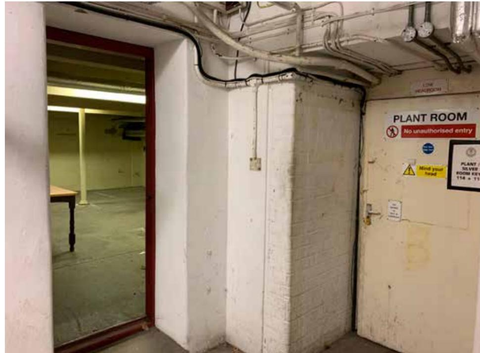
Figure 4.5 A typical corridor within the basement of the hall comprising early nineteenth-century walls which have been inappropriately fitted with exposed MEP equipment. Modern doors have also been introduced here.
