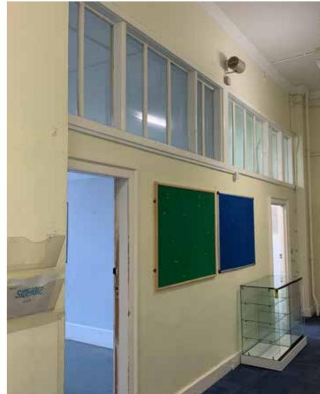
Figure 4.9 Detractive modern partition walls have been installed west of the main entrance hall. They comprise a plain design and have subdivided an historic classroom to create multiple rooms and a corridor
