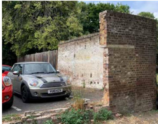
Figure 3.49 Photograph of the surviving section of garden wall. The wall is in a state of disrepair and is structurally unstable
