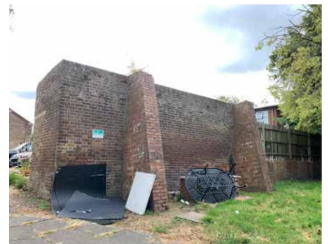
Figure 3.48 The rear elevation of the surviving section of garden wall, showing the modern buttressing. The south returning end of the wall (right) has been rebuilt using modern brick and fencing.
