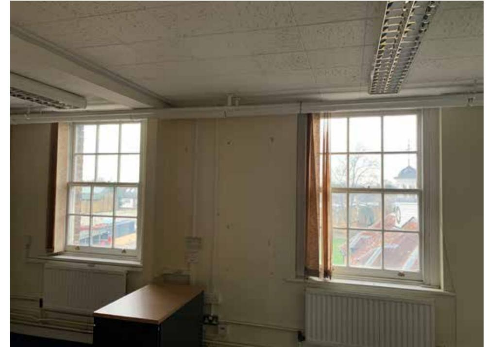
Figure 4.27 A typical modern dropped ceiling located within the west wing conceals the tops of historic windows and negatively alters the historic volume of the space
