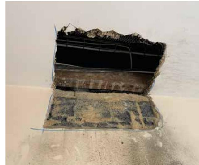
Figure 5.13 Photograph of the heavy block wall build up amongst existing within the west wing at second floor level which are proposed to be removed
