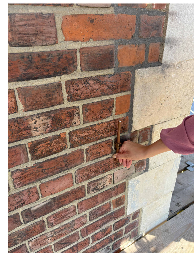
Image 1 Thin copper Lightening Protection tubes dropped down on elevations as per locations on drawing above
