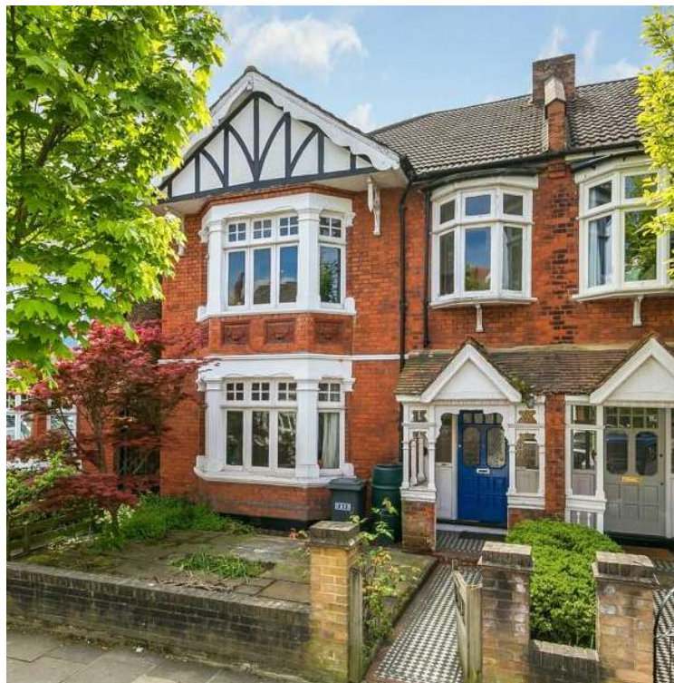
Front elevation of 14 West Park Road
