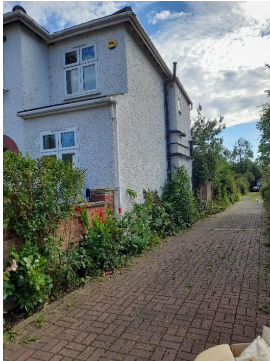
Looking west along drive, number 2 on the left
