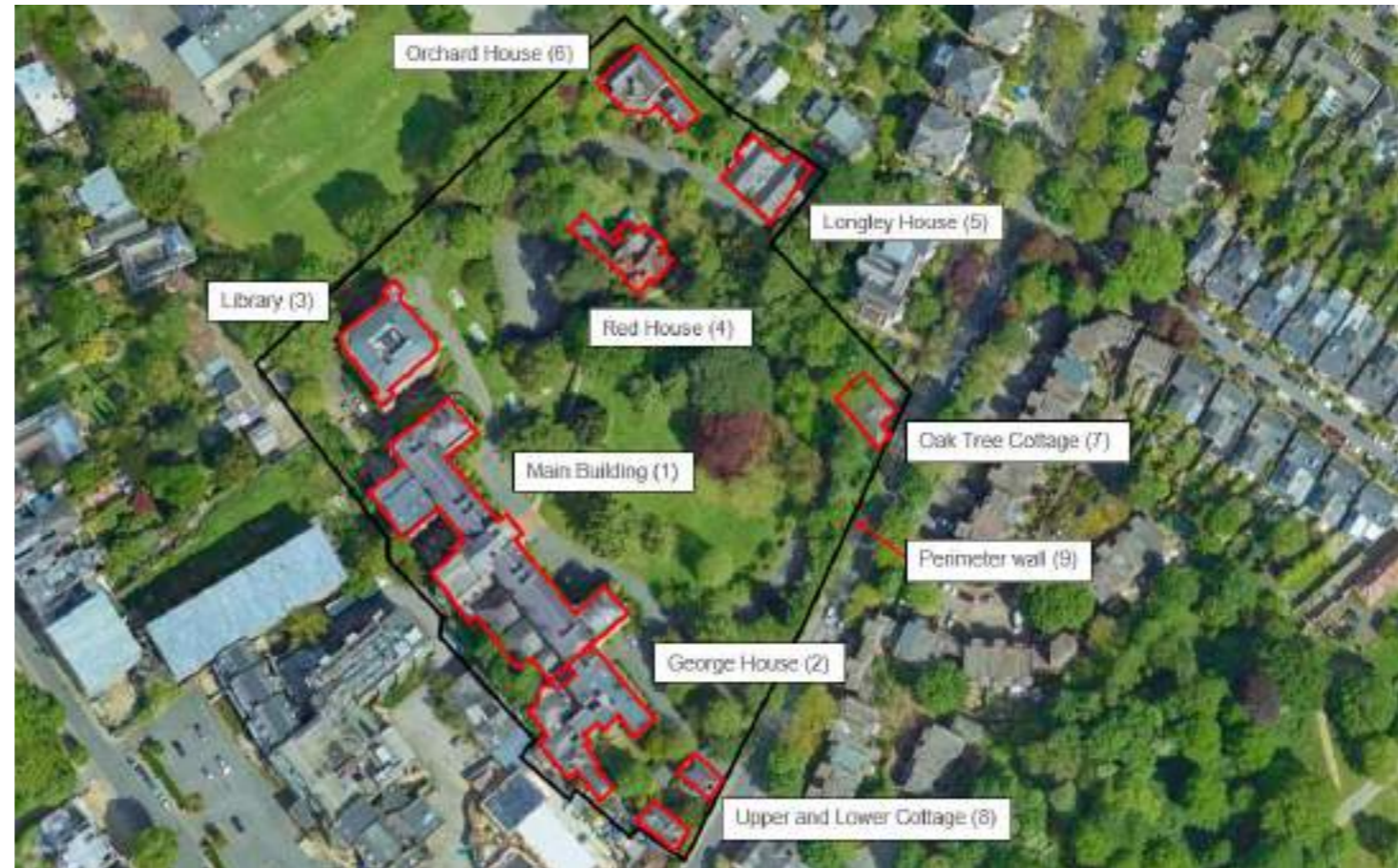
Site overview of existing buildings
