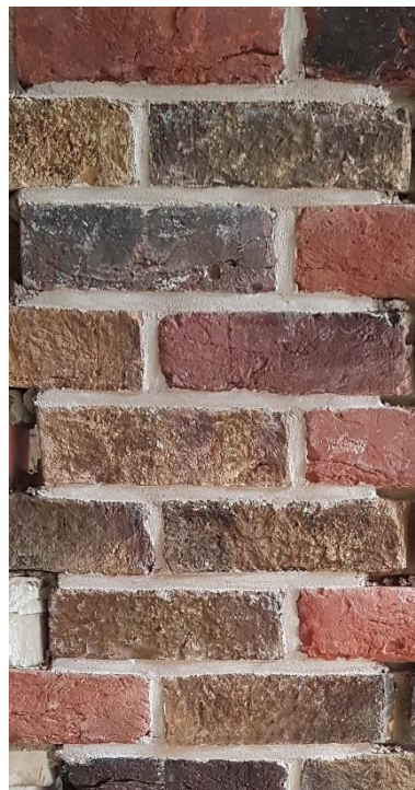
Flush Pointing with lime mortar colour Elm Cragg
