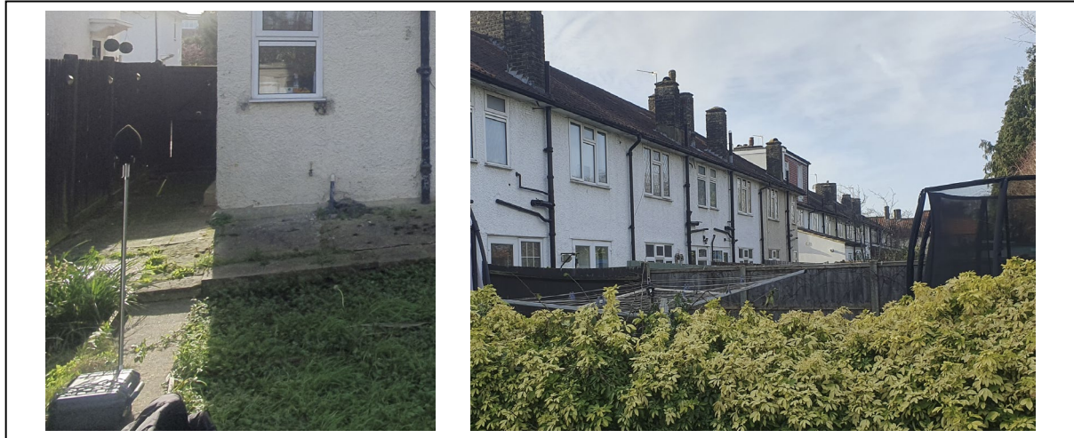
Figure 3: Site Location Measurement Pictures
