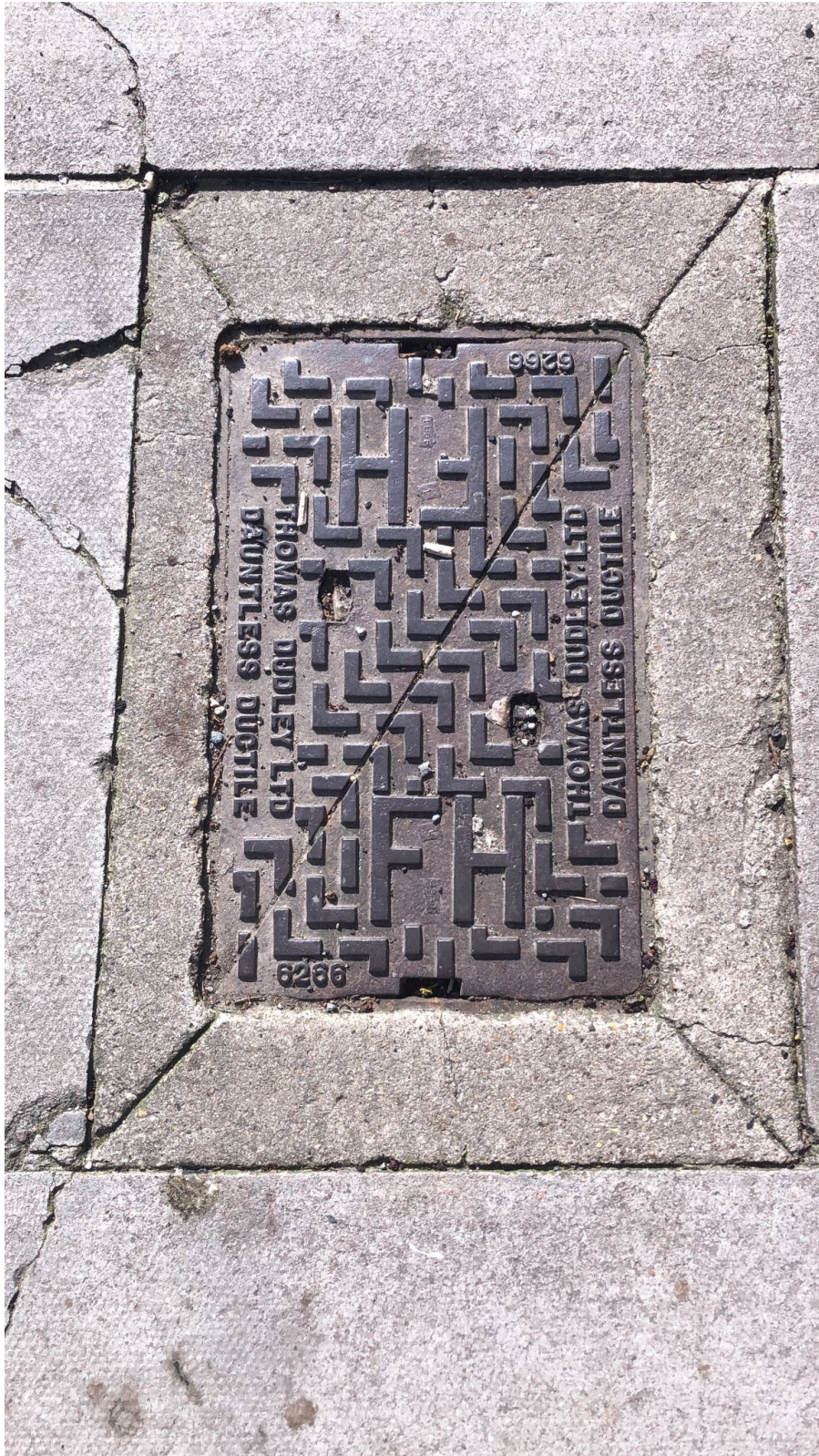
The above photo shows the nearest Fire Hydrant for LFB reference on the opposite side of the road to the property.
