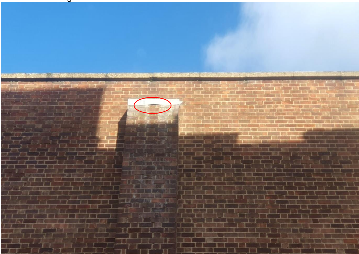
Plate 18: An image showing the gap under the lead flashing on the south-west elevation of the studio building within Block C .
