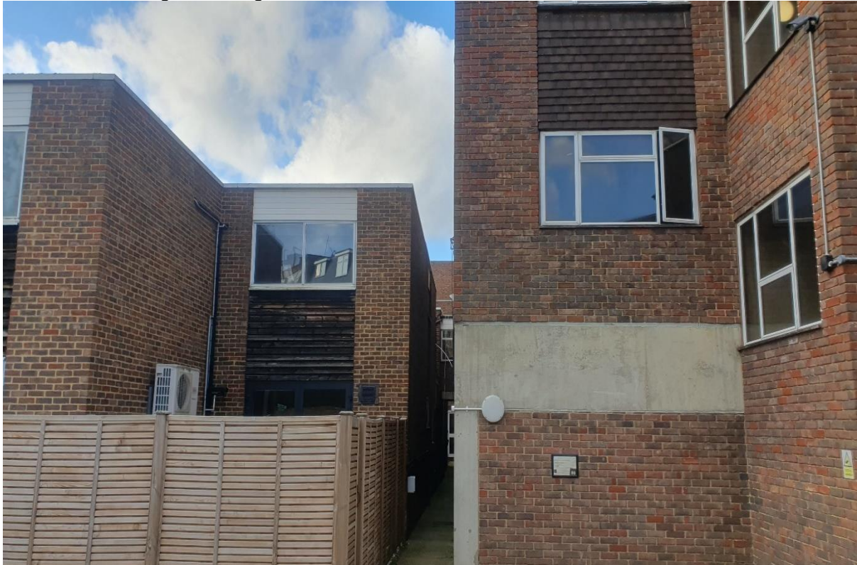
Plate 27: An image showing the south-east elevations of Block H .
