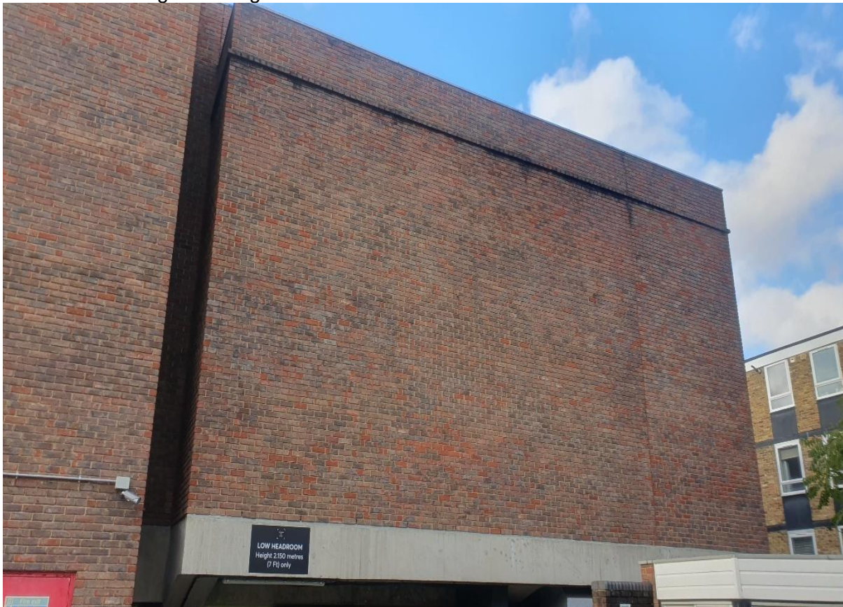
Plate 30: An image showing the south-east elevation of Block H .
