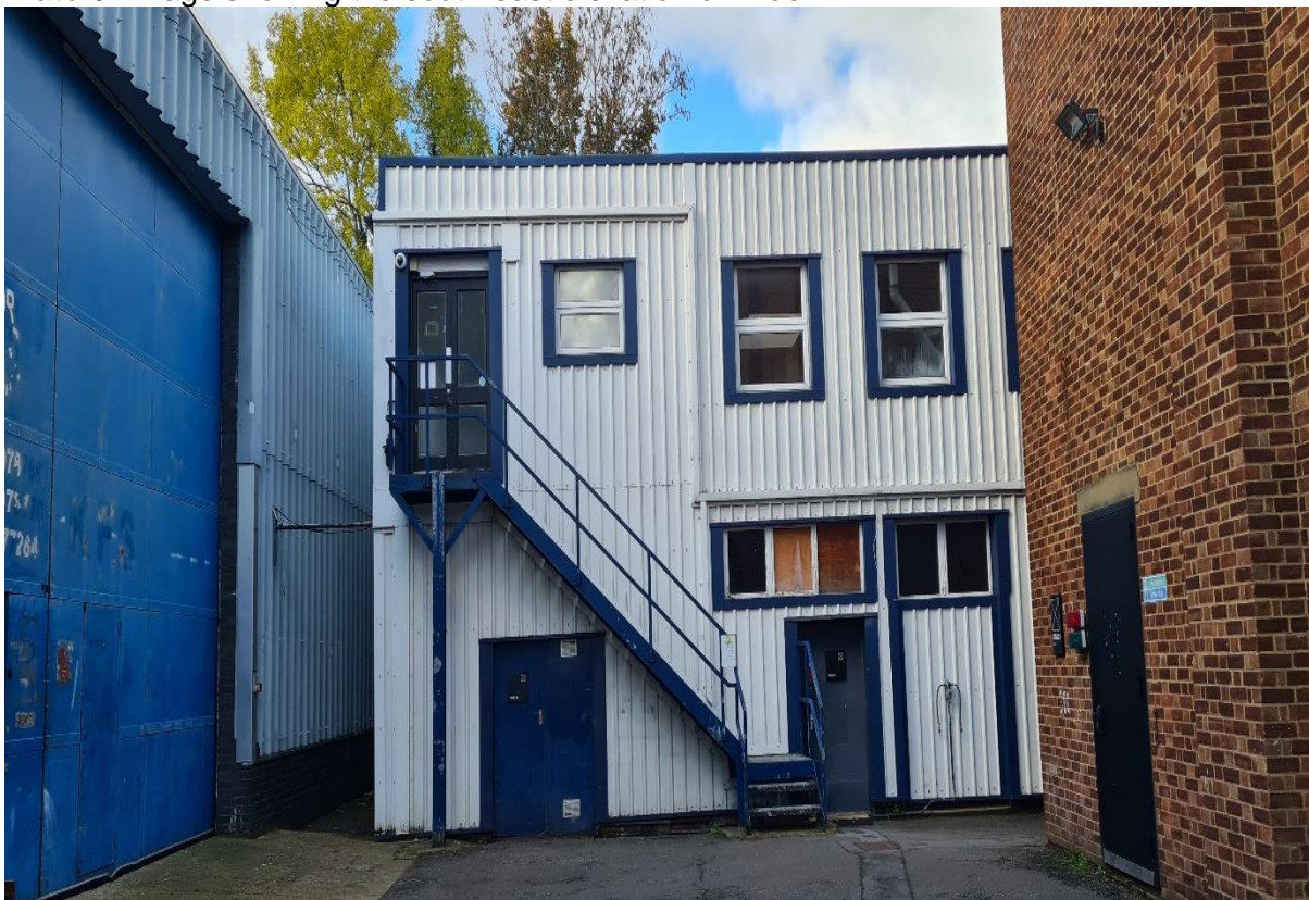
Plate 6: Image showing the south-east elevation of Block D1 .
