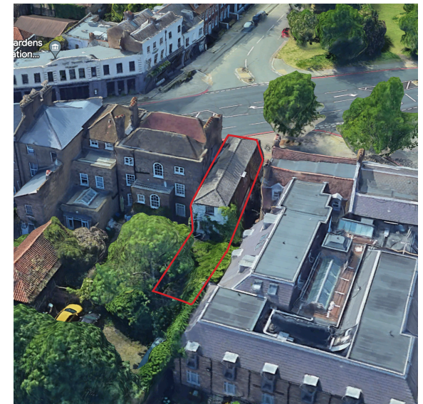
Fig. 4. Google Maps 3D view of rear elevation.
