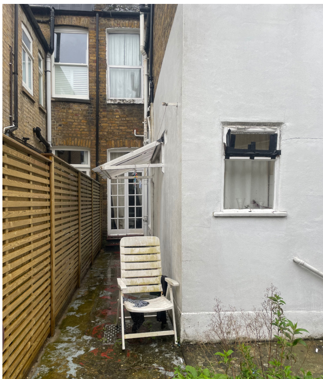
View of rear elevation
