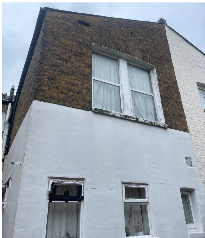
View of rear elevation
