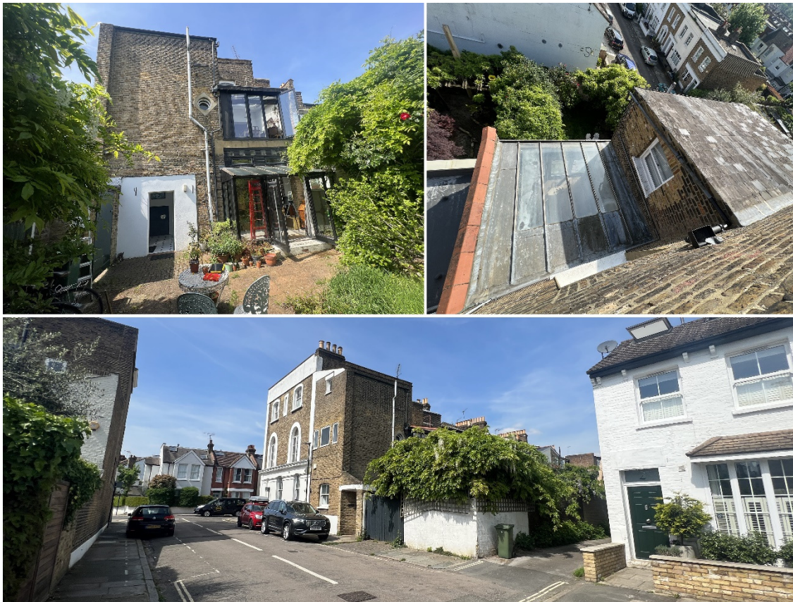
Illustration 3: The existing first-floor rear extension is characterised by outward-swinging doors, which become a distracting feature when open—a frequent occurrence, as this is the only way to ventilate the room. The extension also uses low-quality roofing materials. Additionally, the first and ground floor extensions currently appear as one continuous façade, which detracts from the overall appearance. However, its position at the side of the brick outrigger helps shield it from surrounding views.
