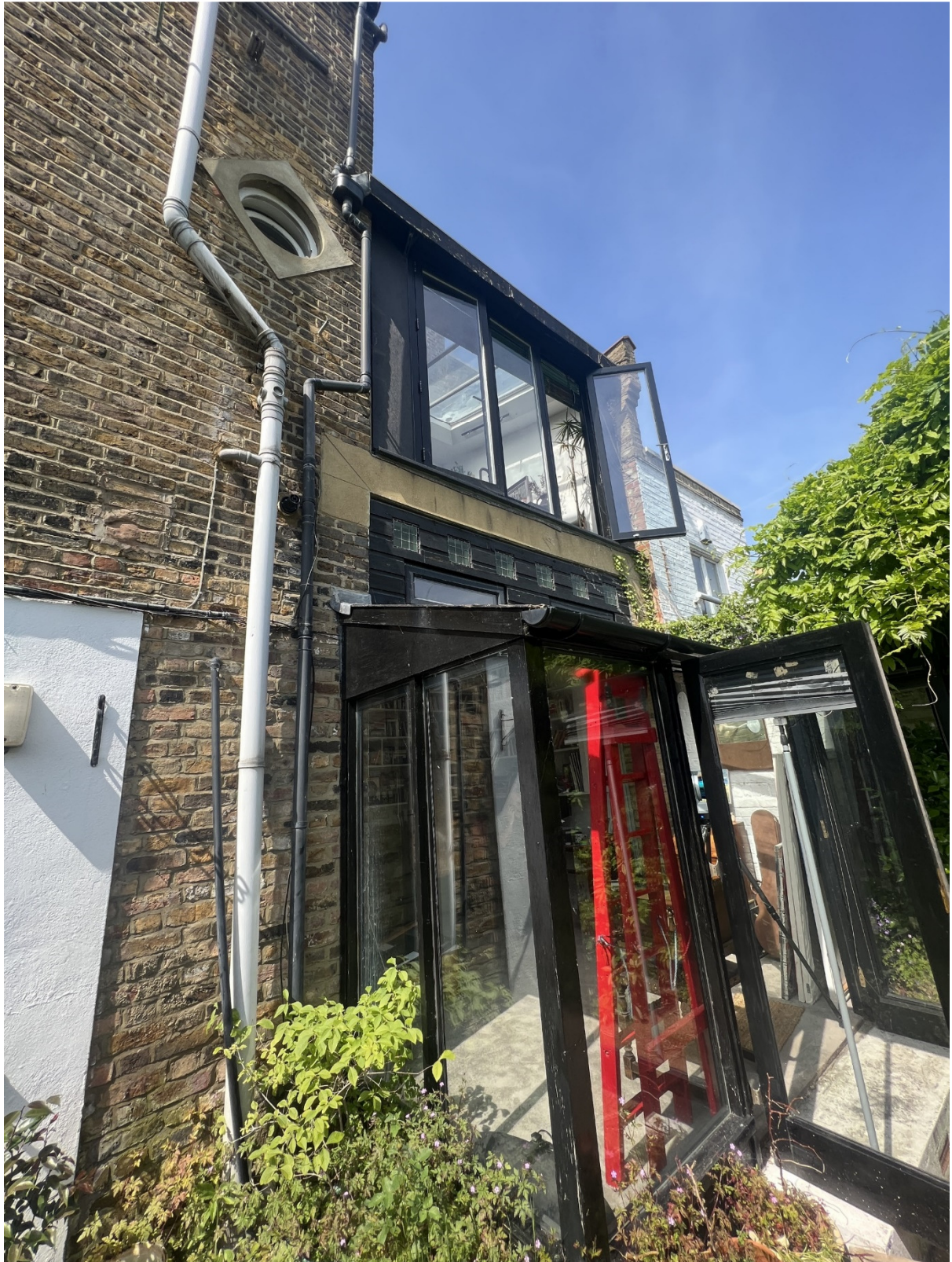
Rear elevation and non-original rear extensions
