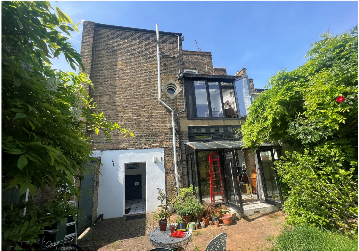
Rear elevation as seen from rear garden
