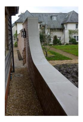
Examples of copings manufactured in cast stone. This is a versatile building material made from aggregates, cement, and natural colour pigments, designed to replicate the appearance of natural stone but achieving uniformity in texture and colour.
