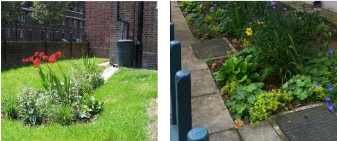
Figure 7 Rain gardens created in Ashby Grove, Islington (left – Susdrain) and at Kingsmead Way, Hackney (right – Groundwork London)
