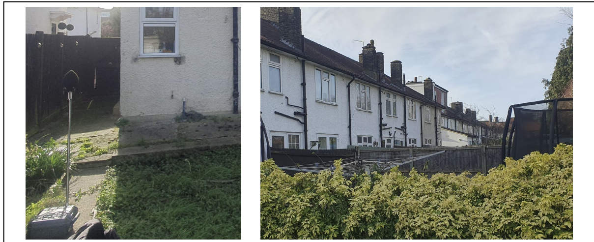
Figure 3: Site Location Measurement Pictures
