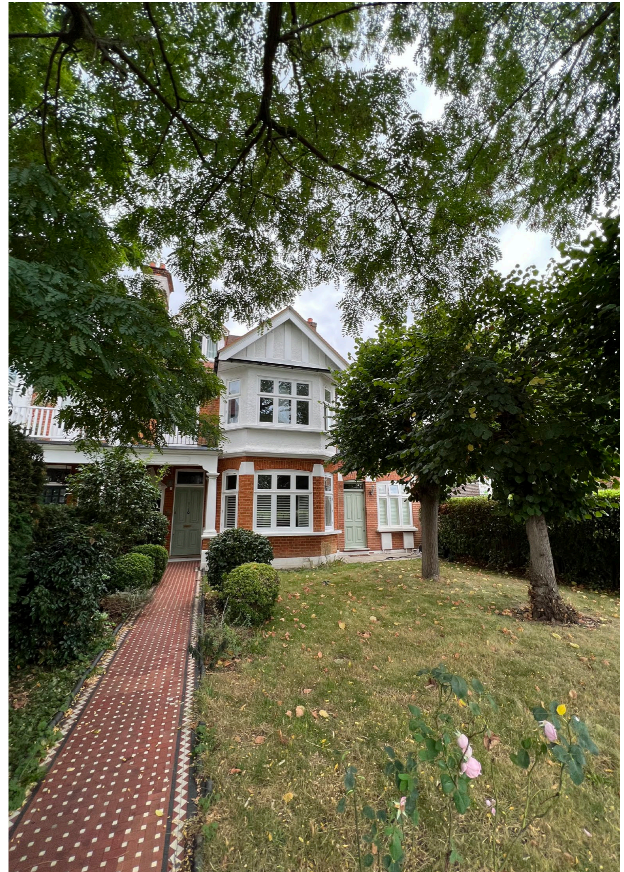
Front Facade from front garden
