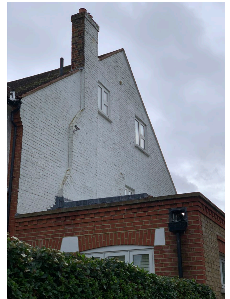
Current side elevation oblique
