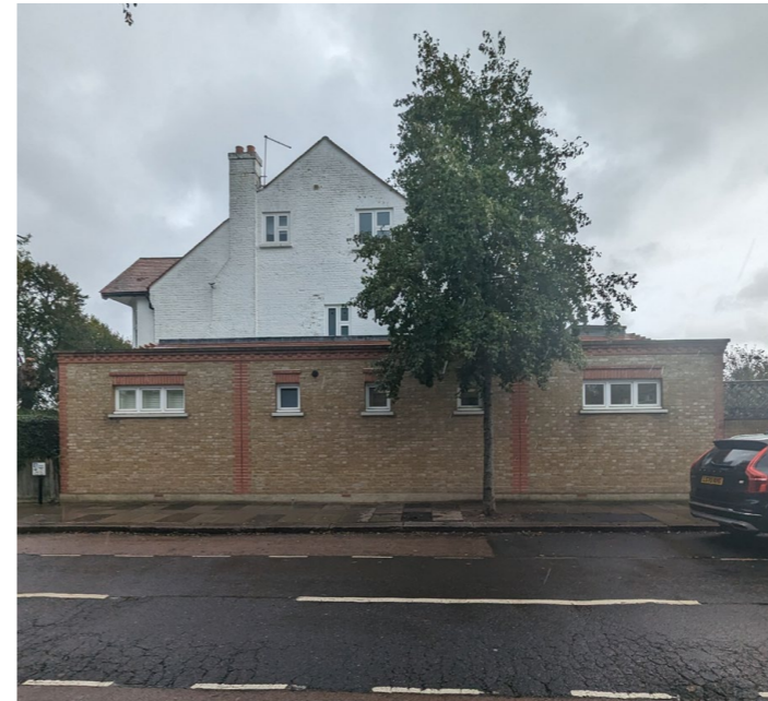
Southwestern elevation along Kilmington Road
