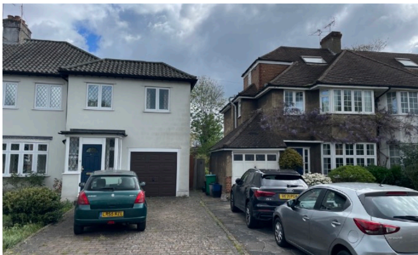
Front elevation No38 and partial No40
