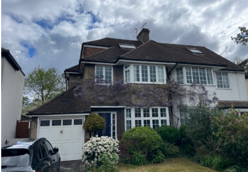
Front elevation No38 and partial No36
