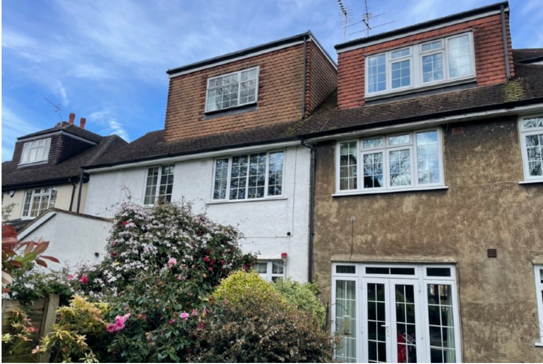
Rear elevation No38 and partial No36
