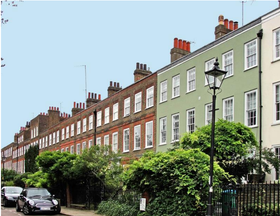
Figure 23 – Front Elevation in context as part of the terrace of Montpellier Row
