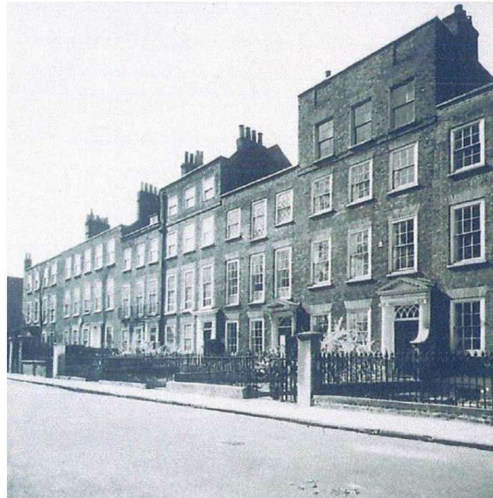
1944 - Photograph of Montpelier Row (not showing Seymour House)
