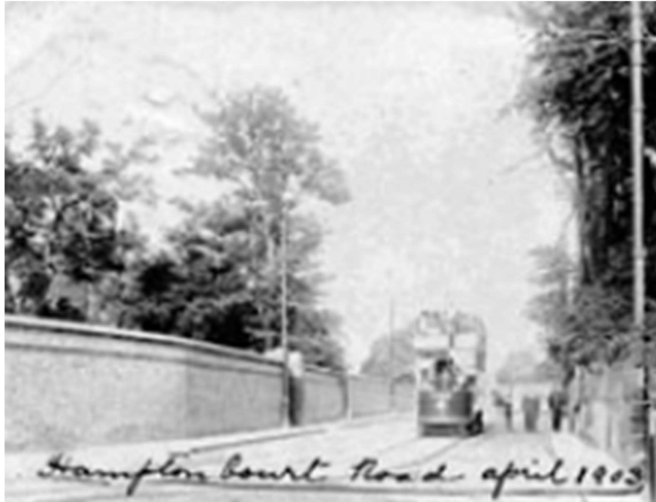
Figure 4: Tram passing Garrick's Villa, Hampton, in 1903 The wall was rebuilt 20 feet inwards to enable the double tracks of the Middlesex tramway route to be built on its new route to Isleworth.
