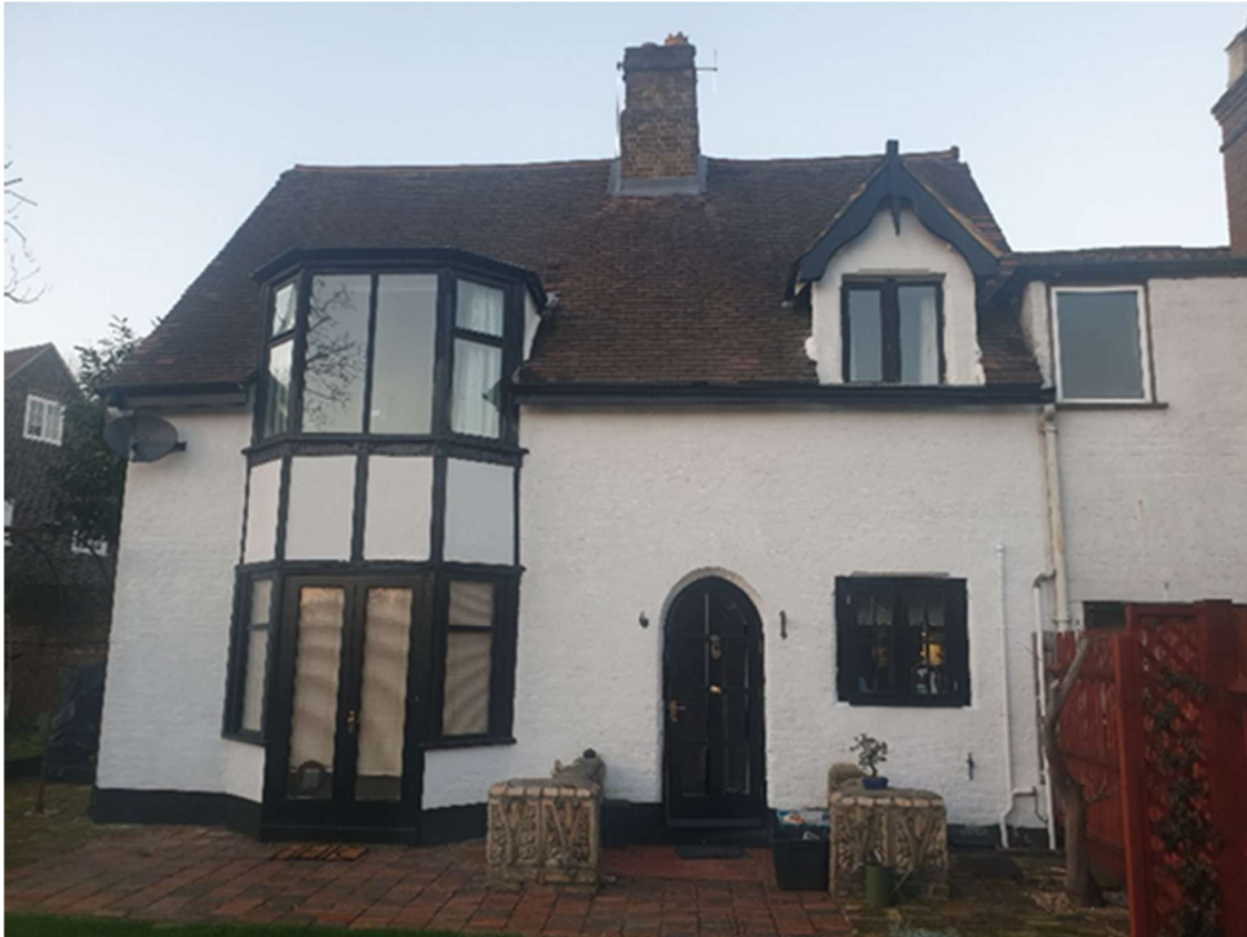
Figure 3 – Front elevation of Garrick Cottage facing Johnson’s Drive: showing non original double height bay window and infill linking element to Garrick Lodge to the right.
