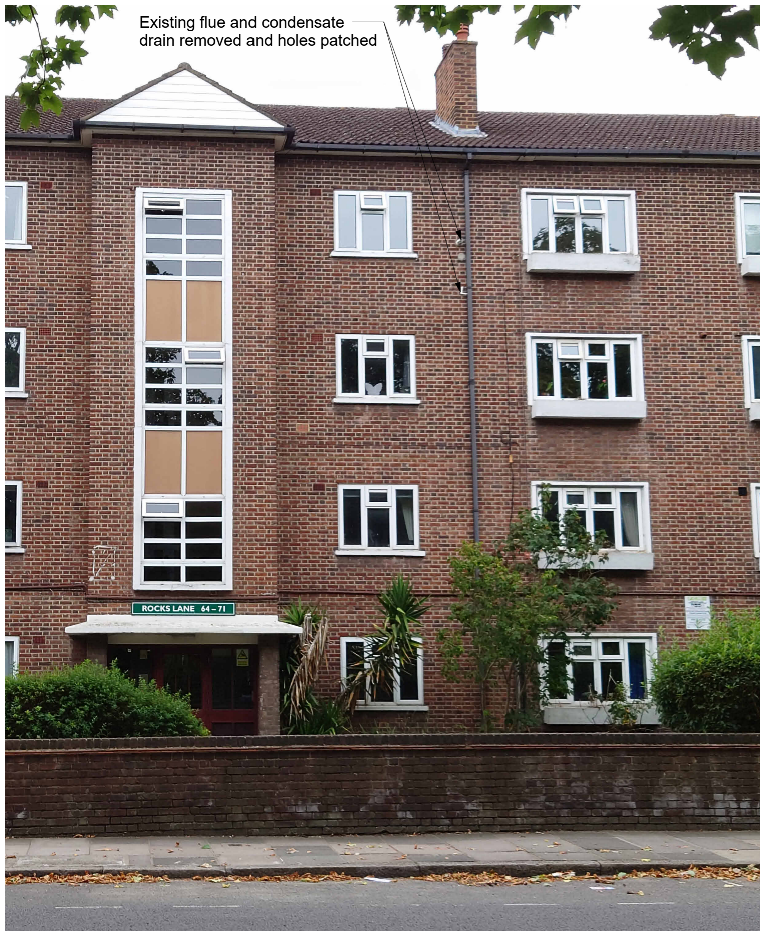
Existing Street-facing East Facade
