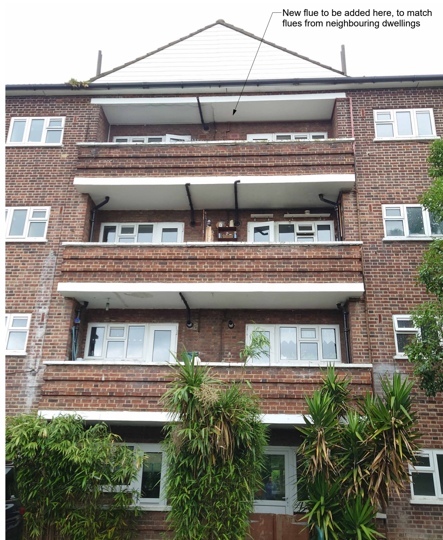
Existing Rear-facing West Facade
