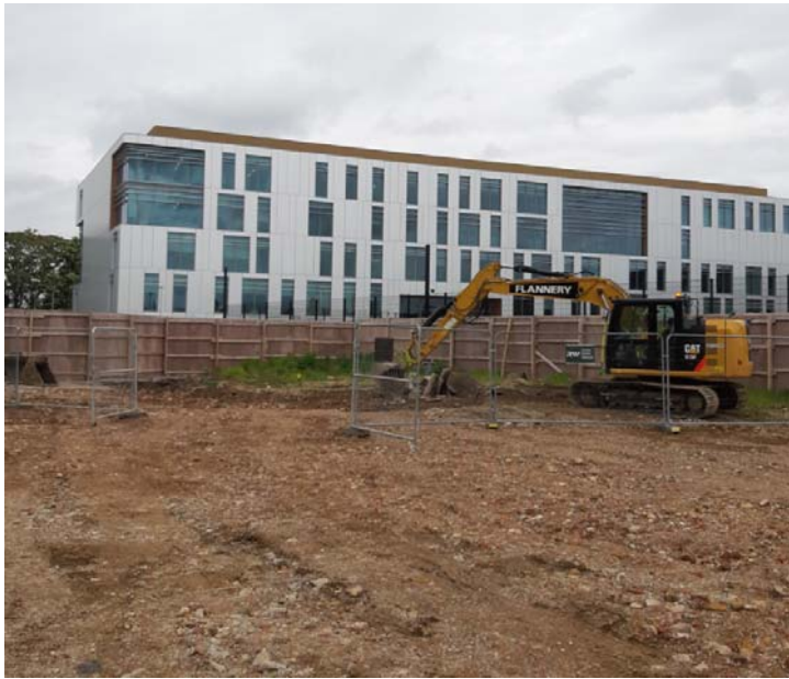
Area secured by RWB ready for in ground chamber removal
