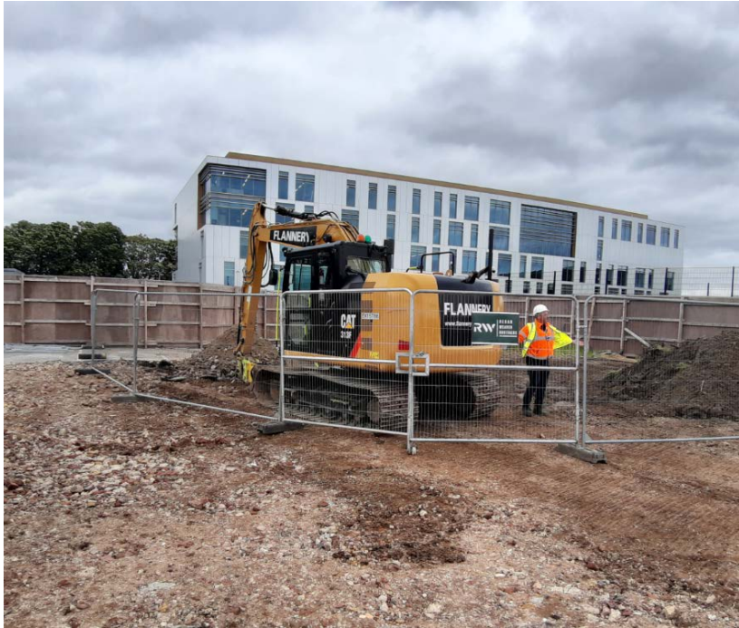
Area secured at end of shift on 20.05.2021
