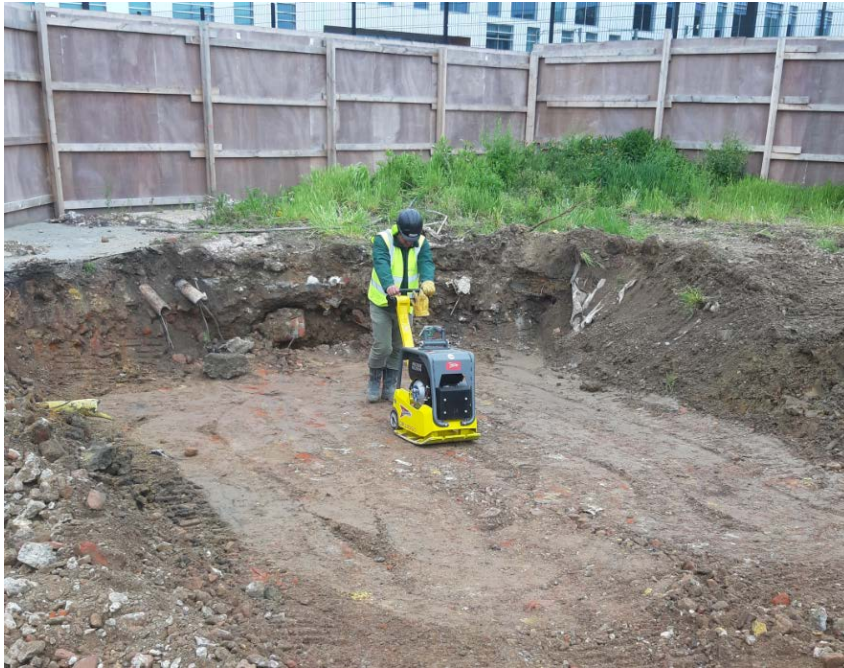
Compaction of backfill to void formed by tank removal
