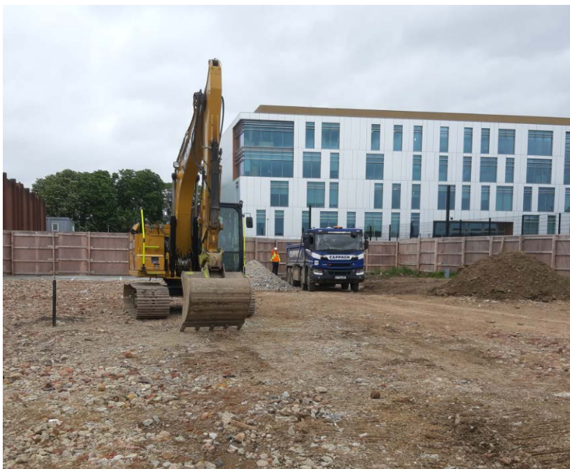
Delivery of backfill material on 21.05.21
