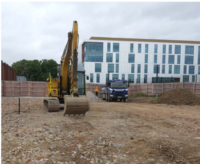
Delivery of backfill material on 21.05.21
