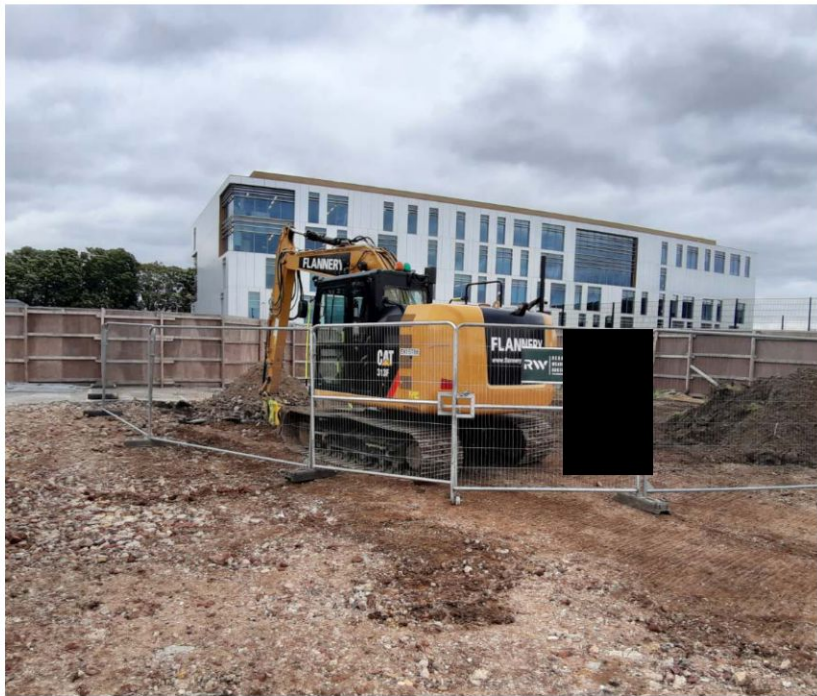
Area secured at end of shift on 20.05.2021
