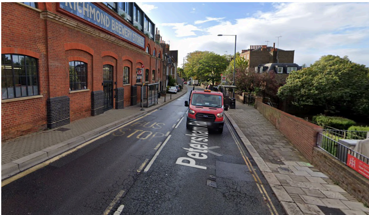
Figure 3-2 View towards site on left hand side
