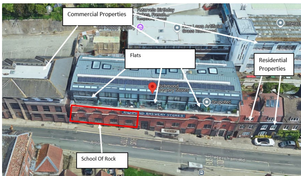
Figure 2: Front facade showing site location and closest receptors
