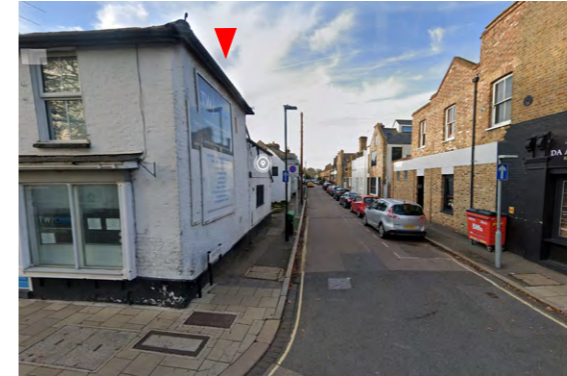
ref.4: View of the Site from The Green frontage.
