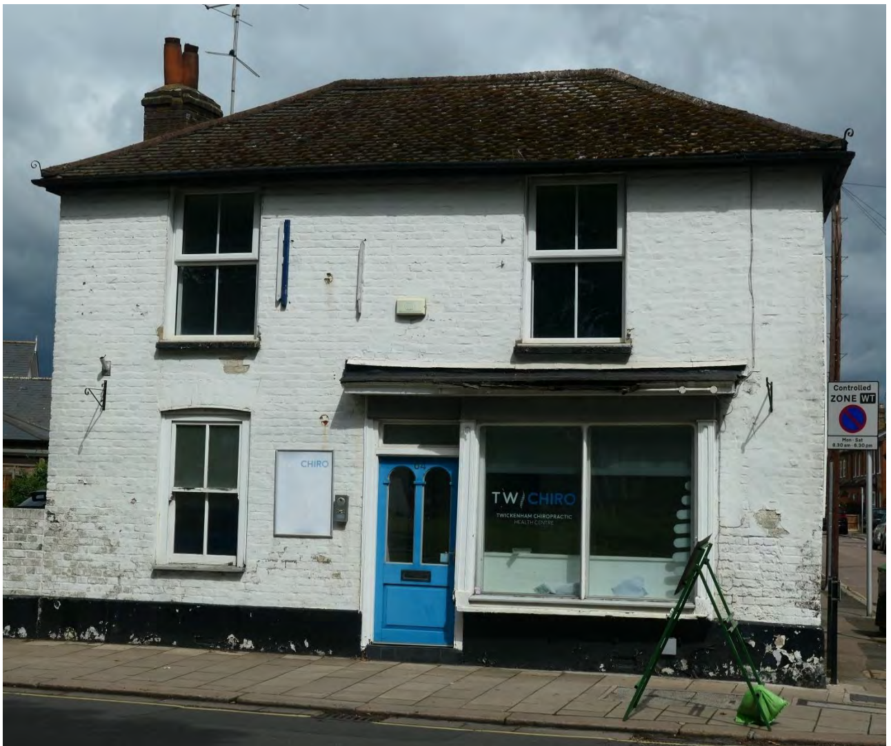
Photo 6: A frontal view of the early C19 corner house.
