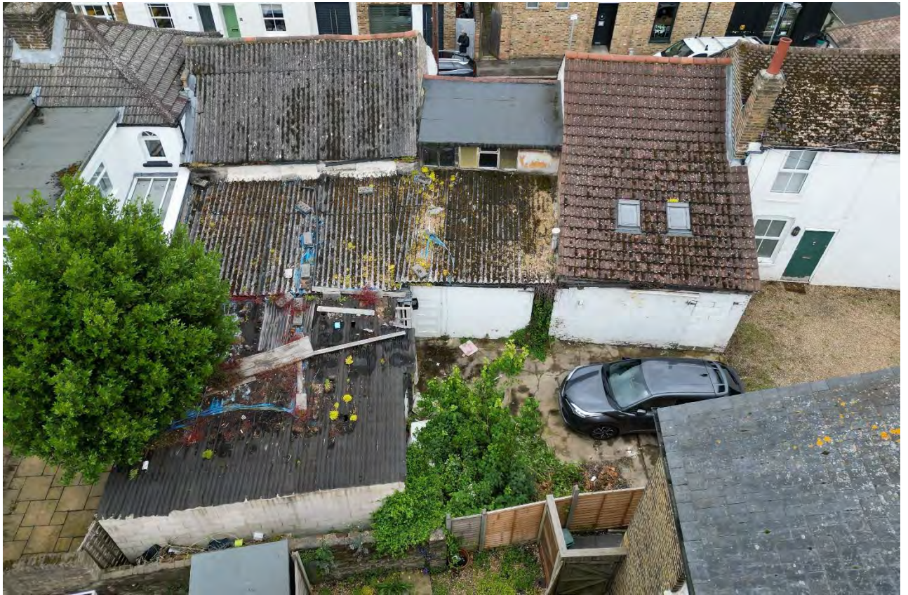
Photo 5: An oblique aerial photo of the application site from the west.
