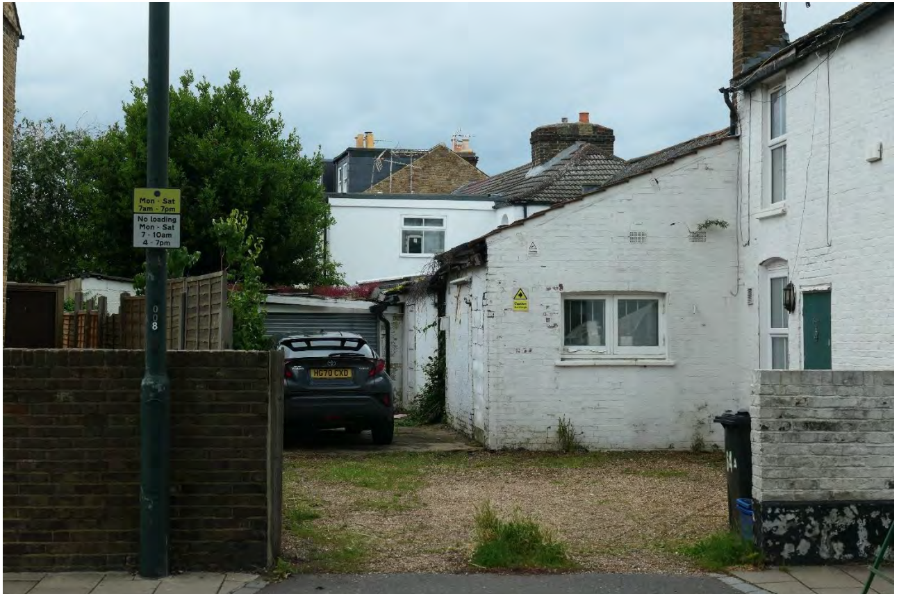
Photo 8: To the west is a short section of boundary wall, with a vehicular entrance that allows parking space for two cars side-by-side on the gravel surfaced area; beyond this, the largely modern and very poor quality piecemeal and had hoc accretions to the rear 'workshops' can be seen.
