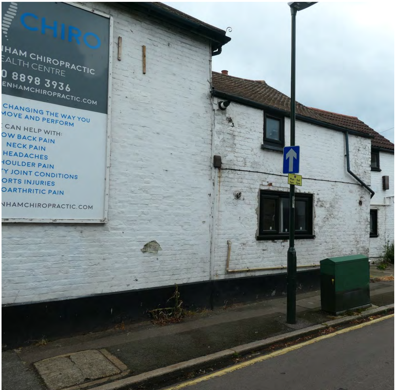
Photo 9: The east return elevation of the early C19 corner house and the catslide infill on May Road.
