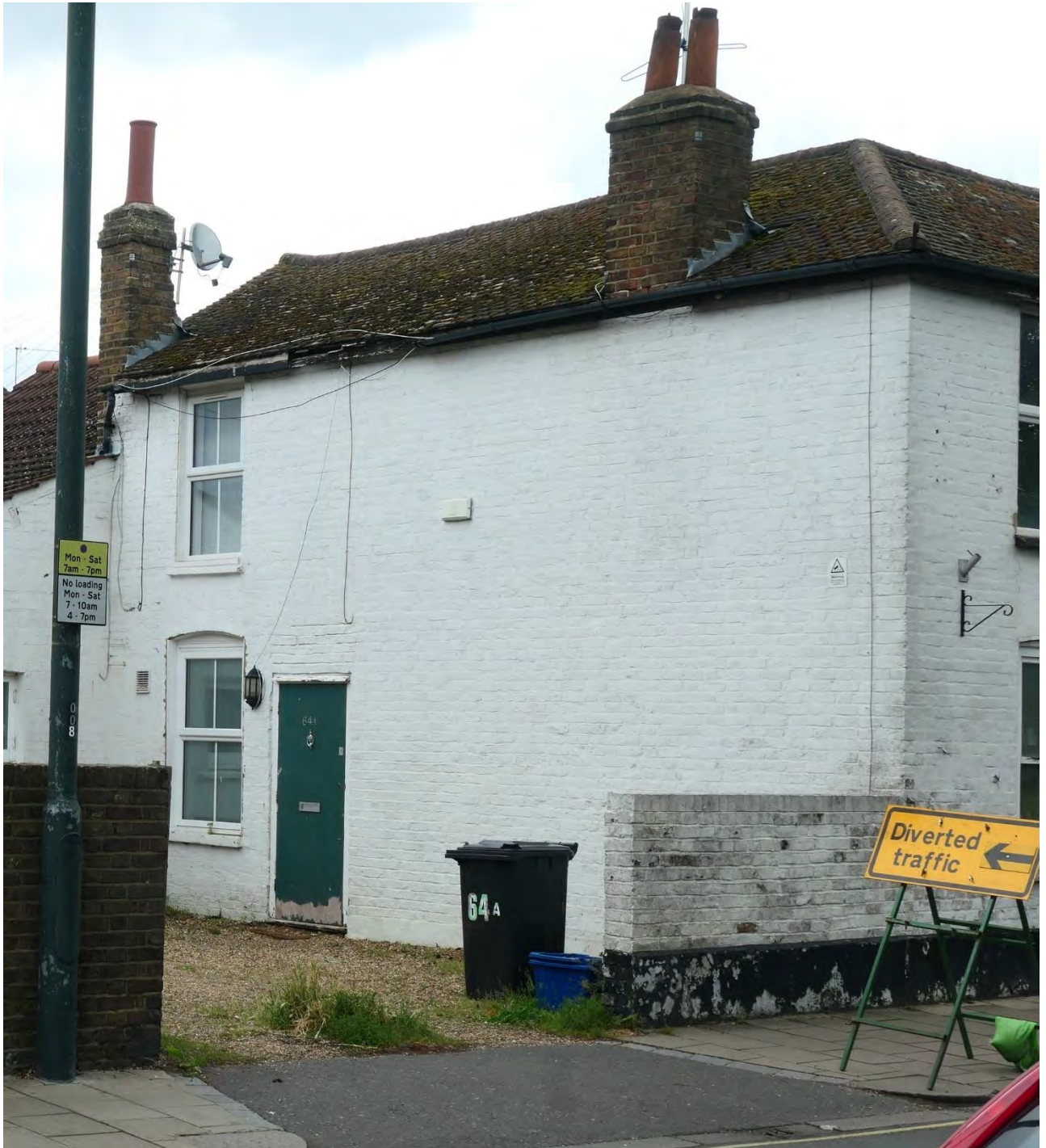
Photo 7: The west return elevation (Photo 7) is largely blank, aside from an inserted modern door and a set of windows at the northern end. It is not an especially notably part of the building for any reason.
