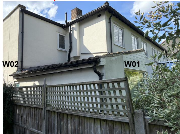
PIC 01 showing W01 and W02
