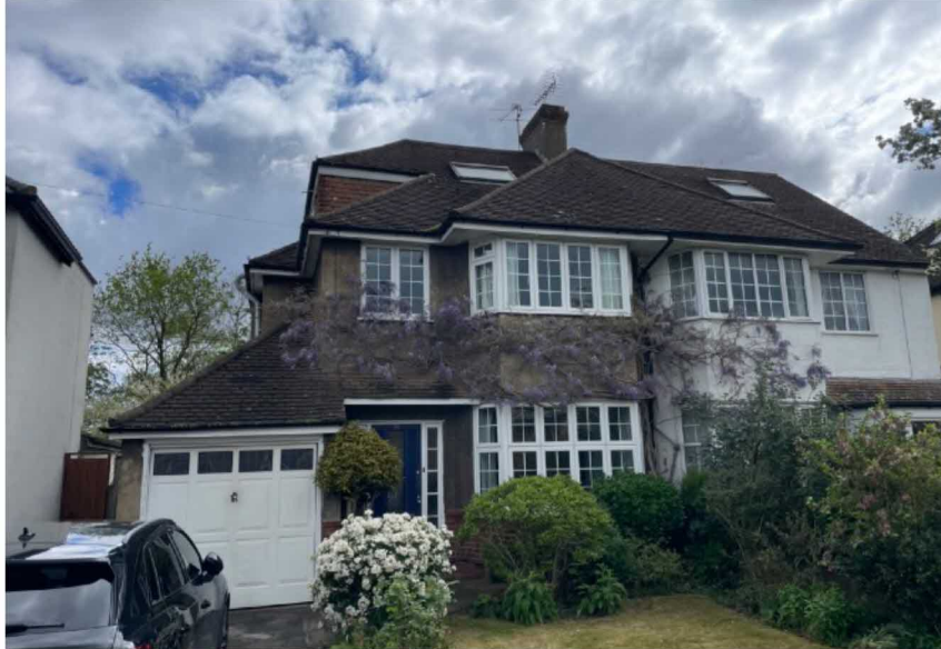
Front elevation No38 and partial No36
