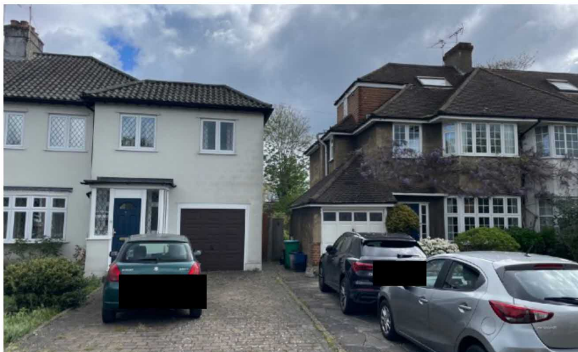
Front elevation No38 and partial No40
