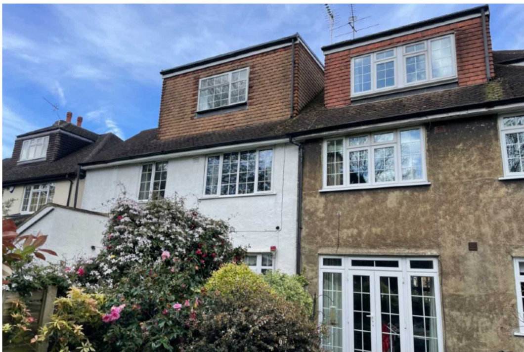
Rear elevation No38 and partial No36
