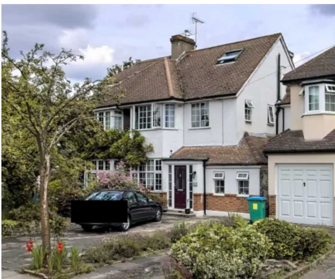
Porch at No36
