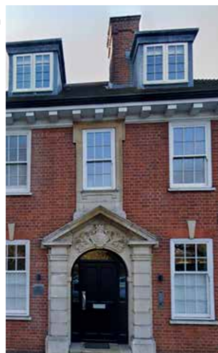
Cambridge House, 15 High Street - stone details and red brick
