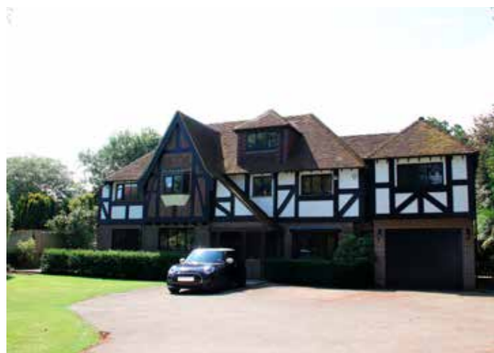
Front view of the existing house
