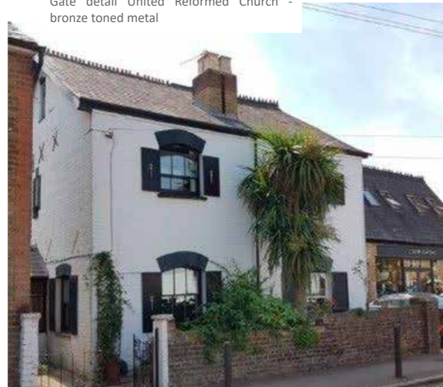
1-3 Windmill Road - timber shutters and neutral toned rendered brick. Grey brick wall along pavement.
