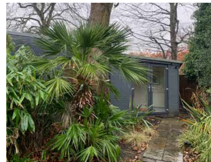
View of approach from rear garden to outbuilding 2
