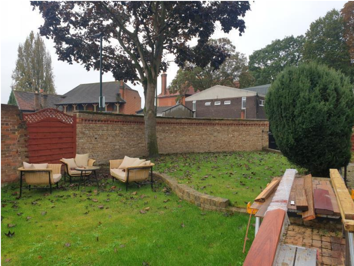
Figure 8: Looking south-west towards the dwarf wall within the garden area adjacent to T3 (centre), showing also the area of the southern brick boundary wall to be in-filled.
