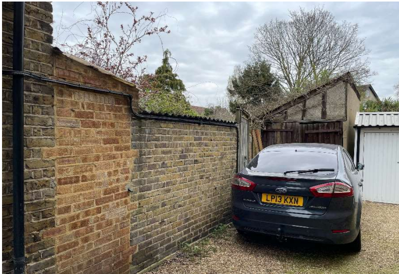
Existing garage and side wall enclosing garden from drive
