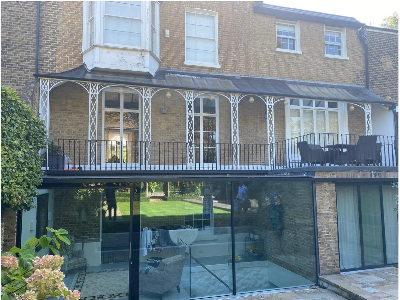
Figure 7 – Rear elevation, 107 Castelnau.
